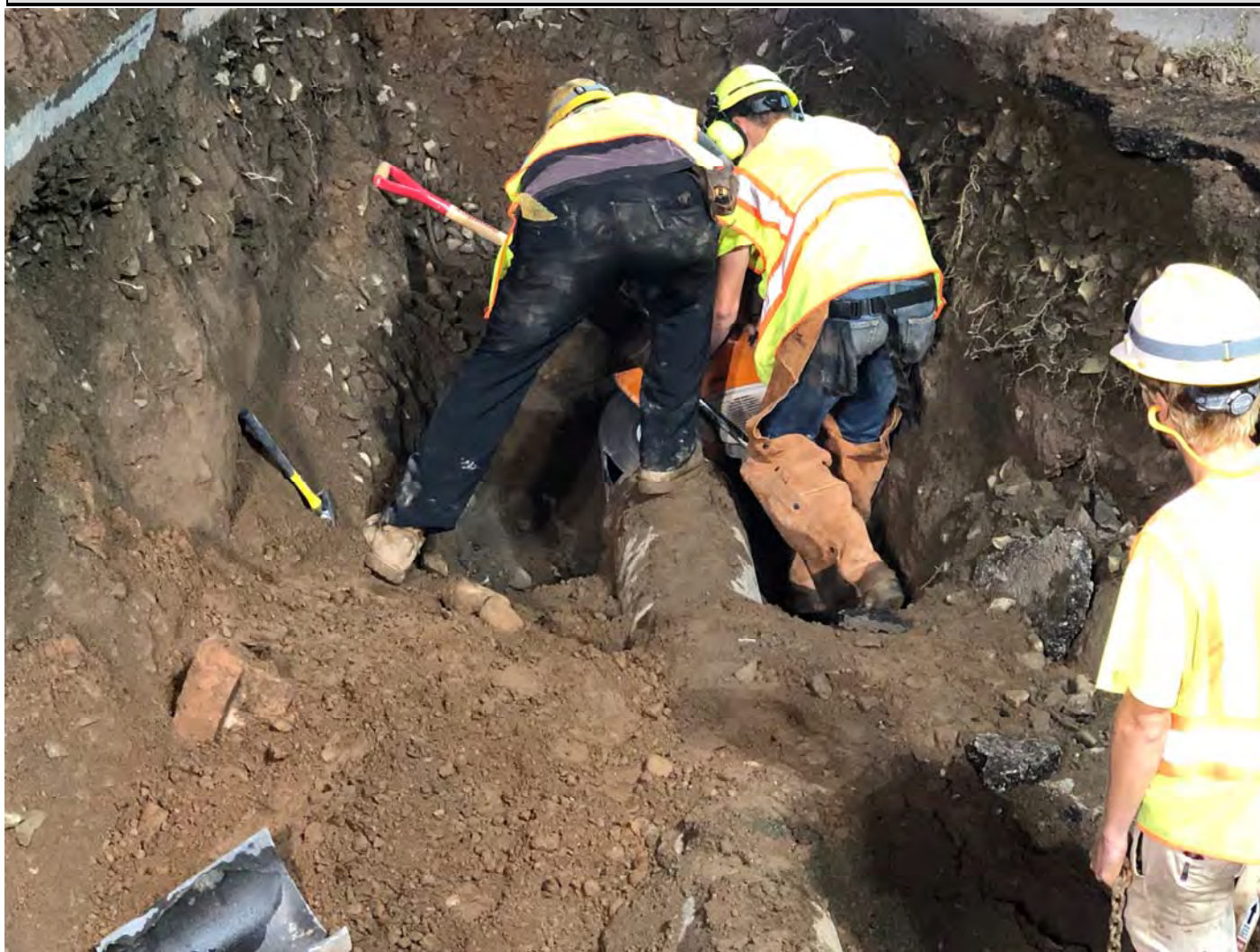
Figure 4 – Making second cut into existing water main
