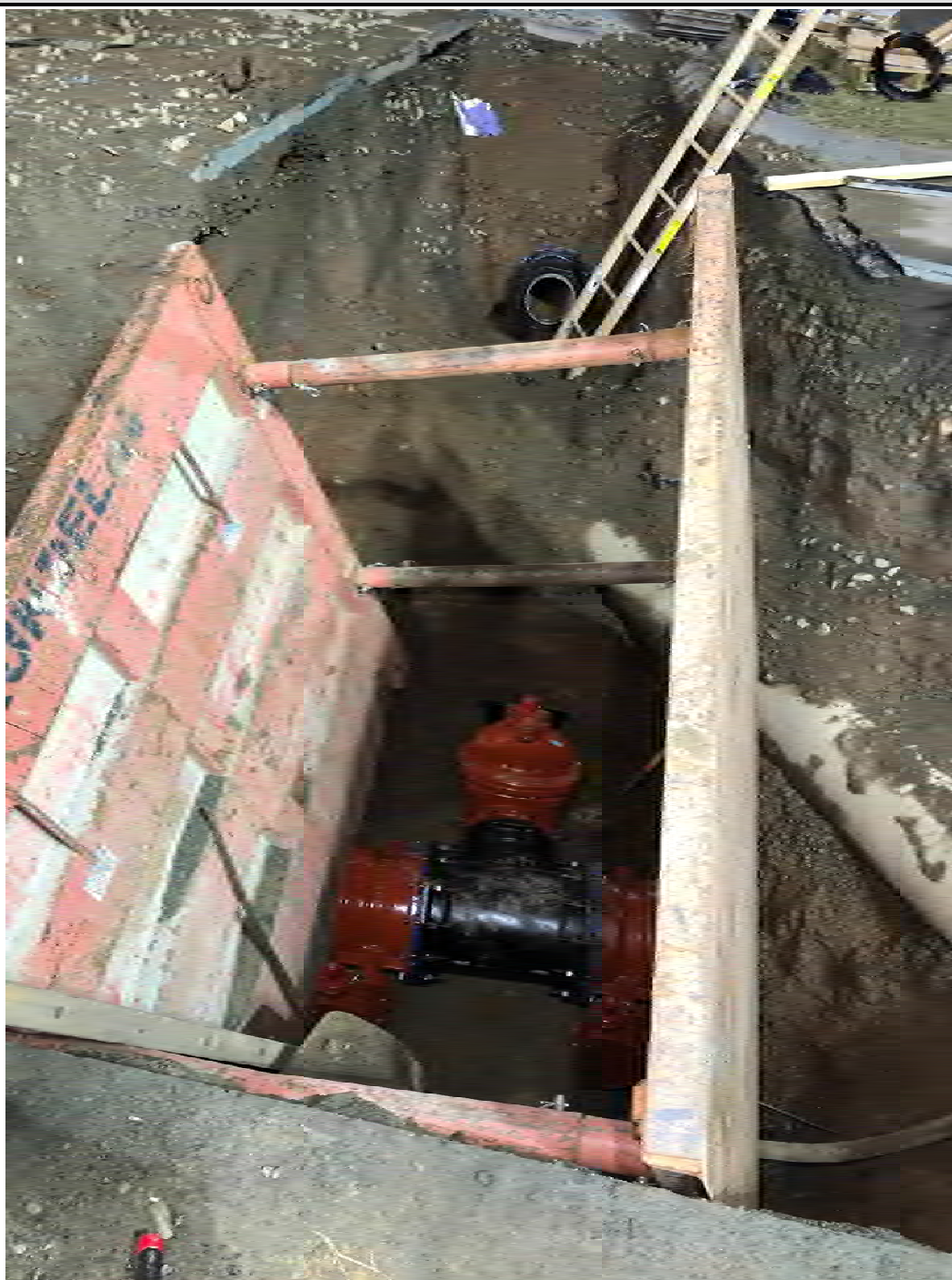
Figure 8 – Tee and valve section in place in trench
