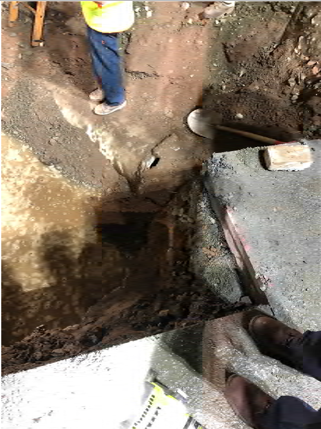
Figure 3 – Hole in existing storm drain pipe
