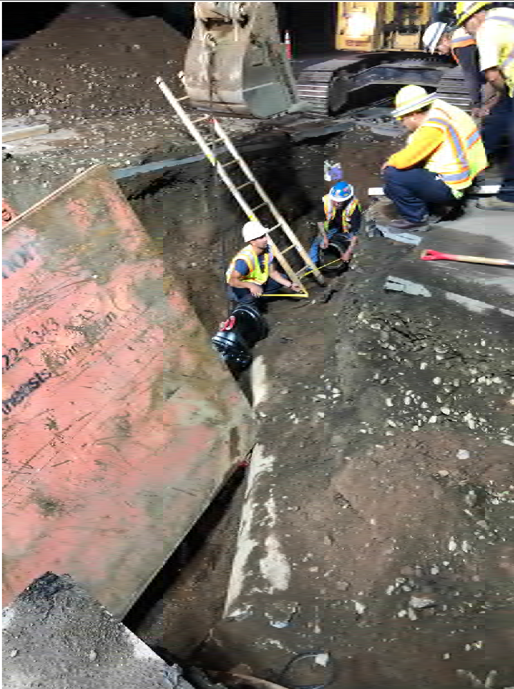
Figure 10 – Measuring length of pipe needed to connect upper 45-degree vertical bend to the existing water main
