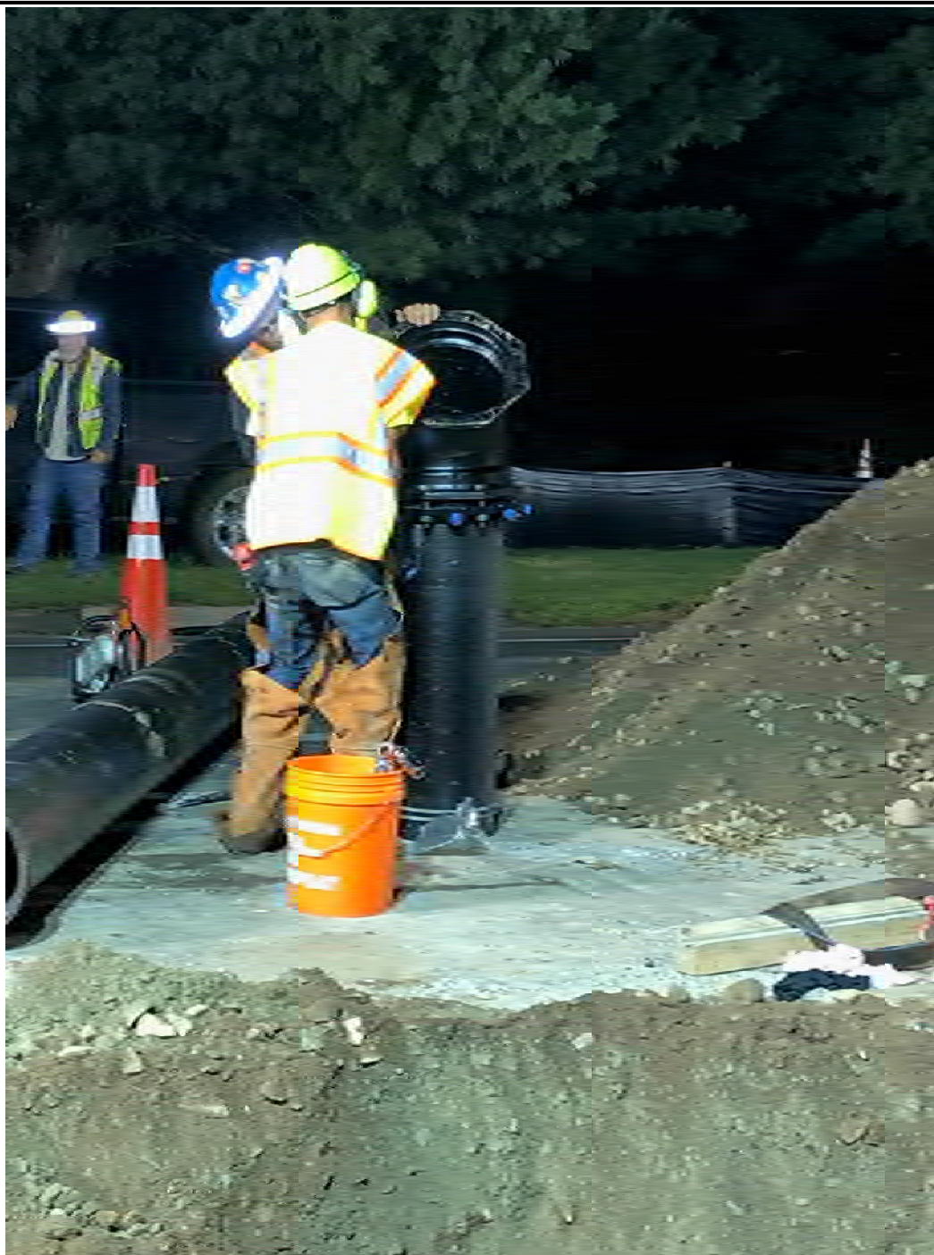
Figure 7 – Assembling connections for the 45-degree vertical bend section
