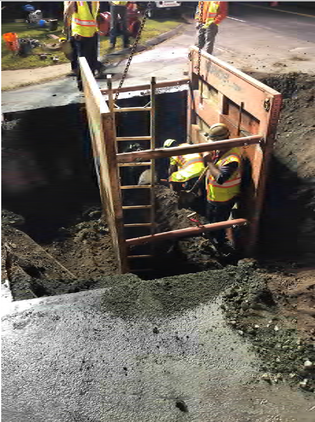
Figure 2 – Making first cut into existing water main
