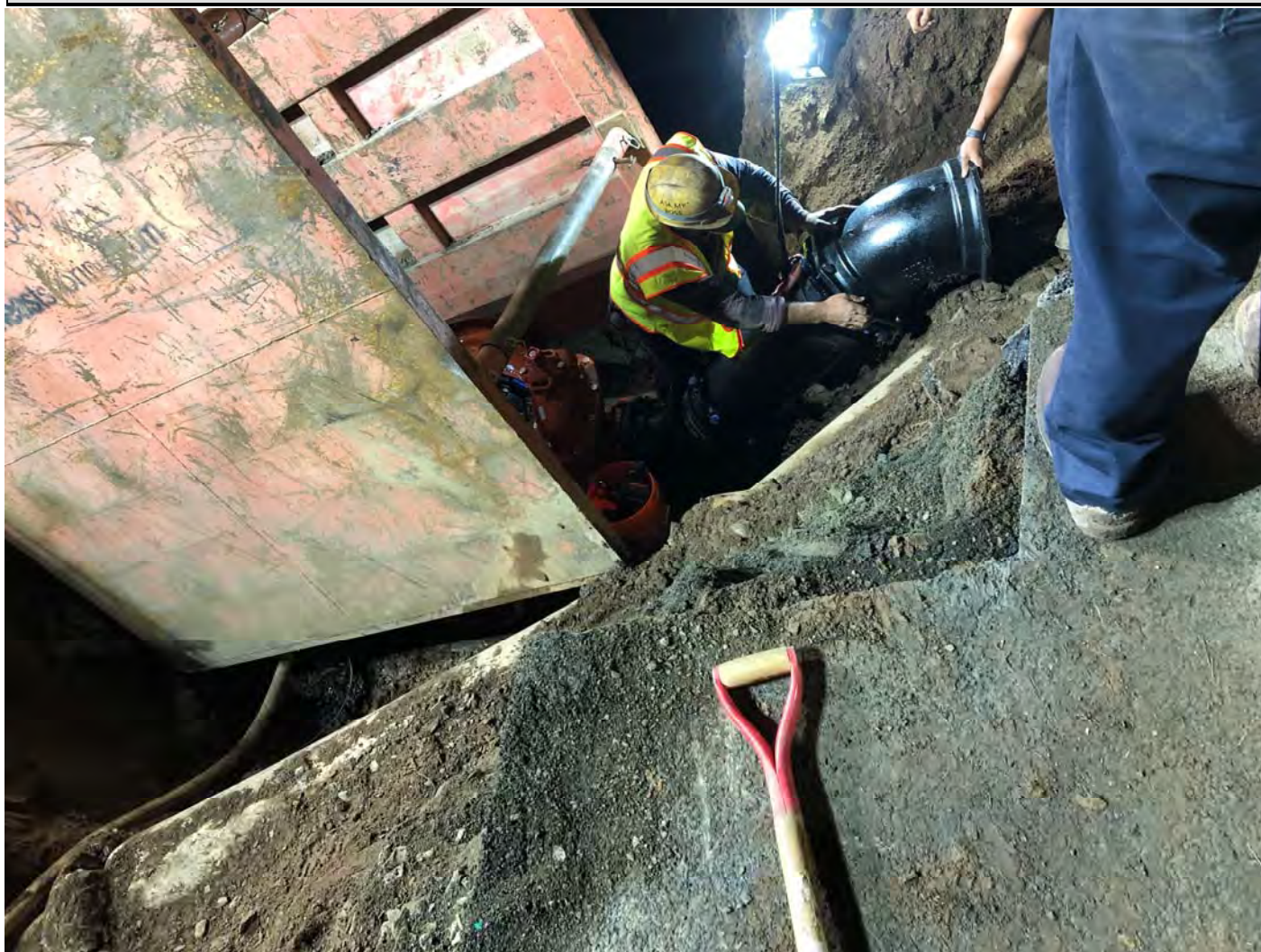
Figure 9 – Attaching connector piece with 45-degree vertical bend to the Tee section
