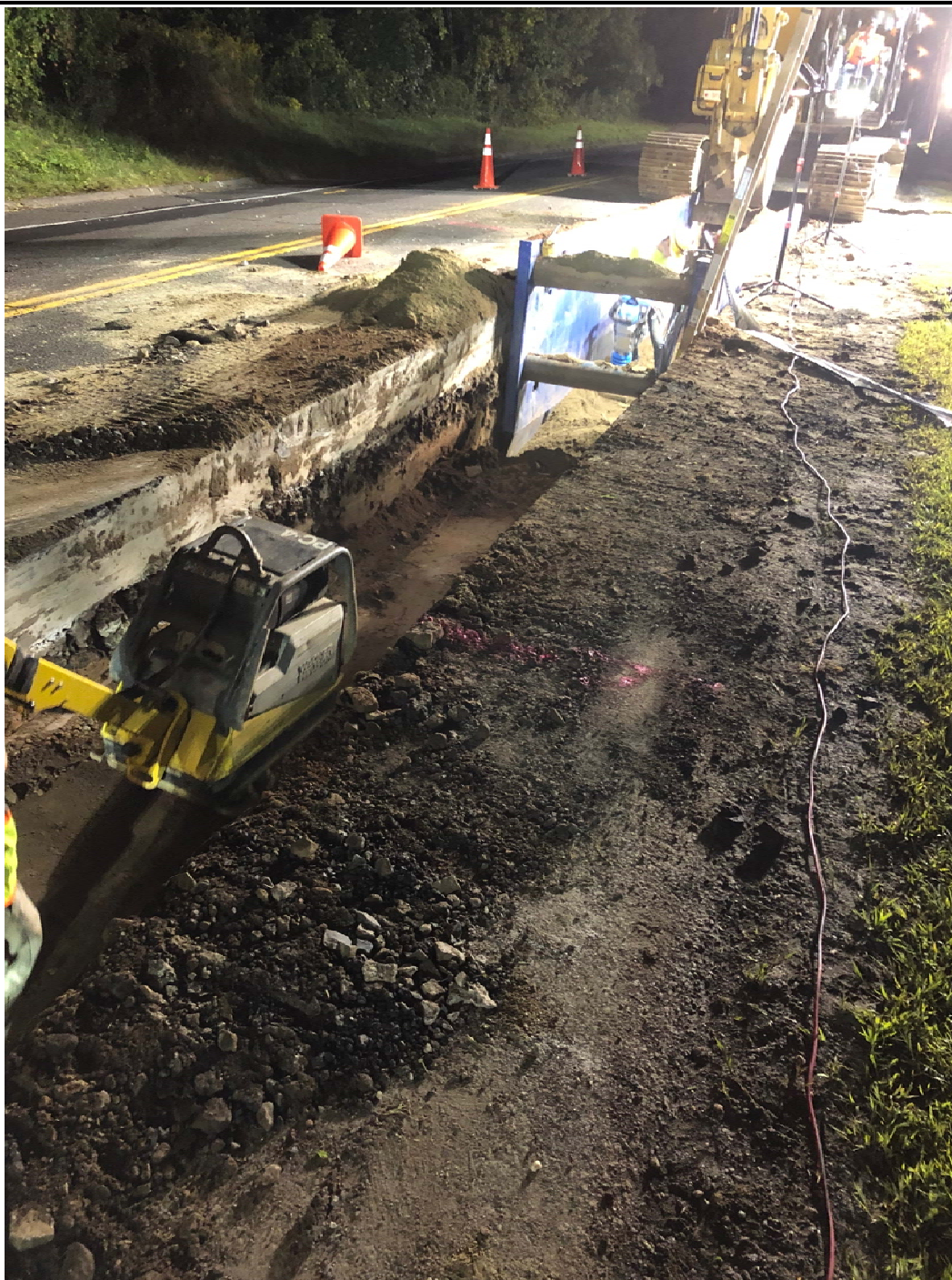
Figure 1 – Compacting 2 nd fill layer above 2 nd , 3 rd pipes and compacting 1 st fill layer above 4 th pipe
