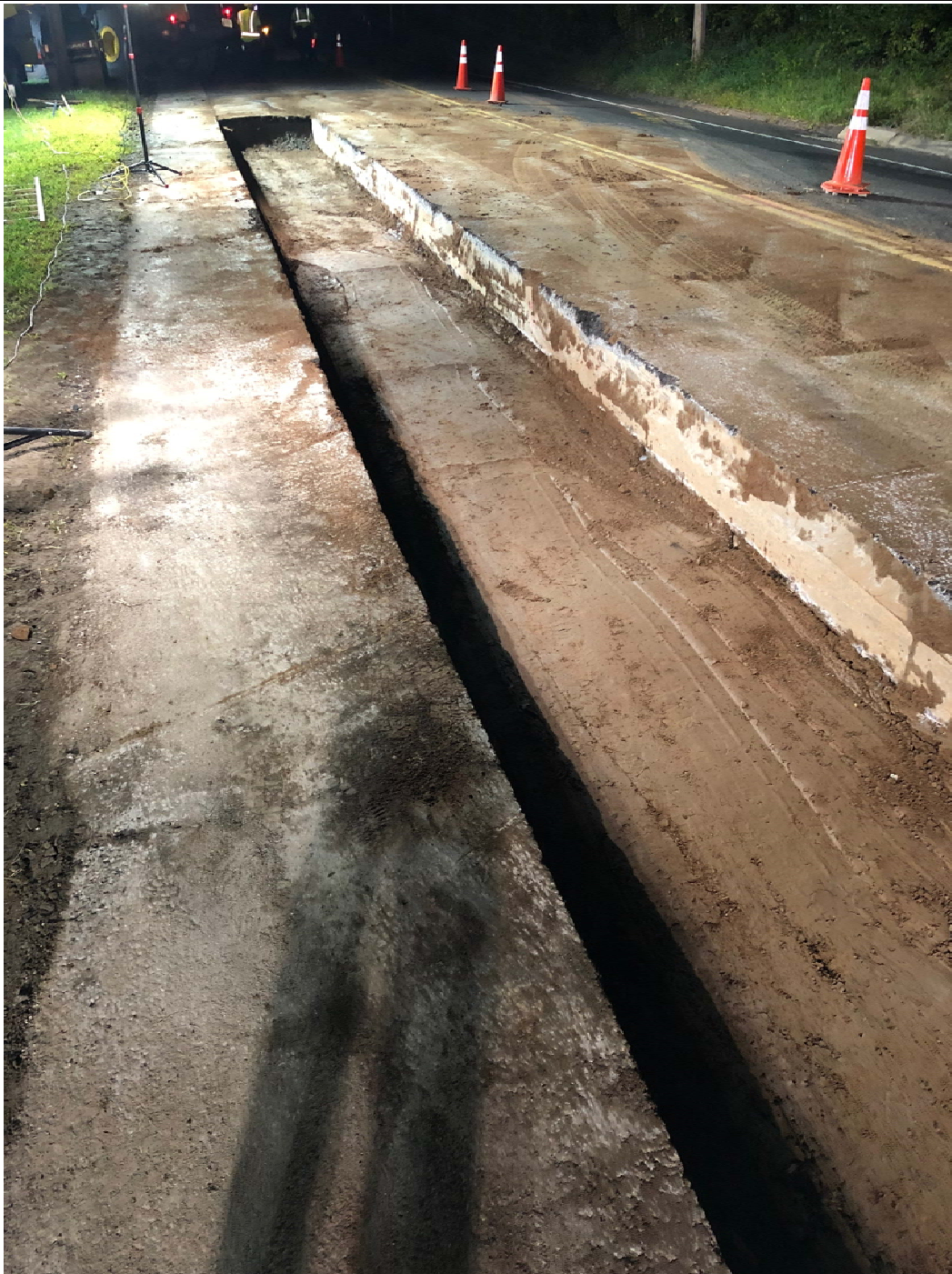
Figure 2 – Compacted fill above 1 st -4 th sections, ready for processed stone layer
