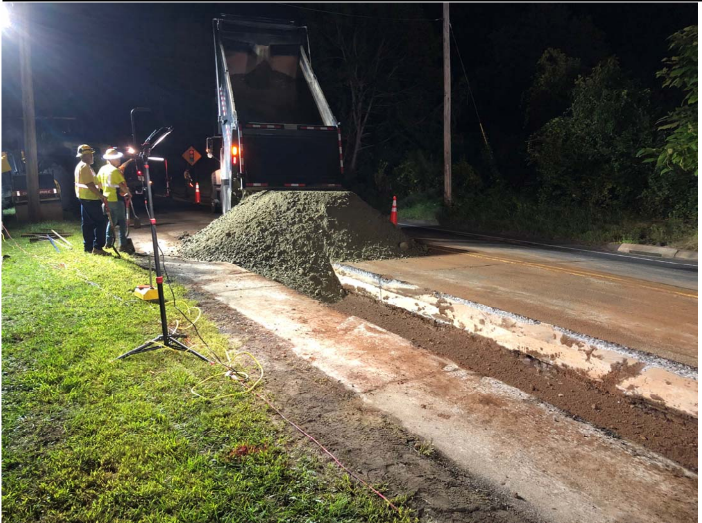
Figure 3 – Processed stone being dumped, preparing to be graded with road in the trench
