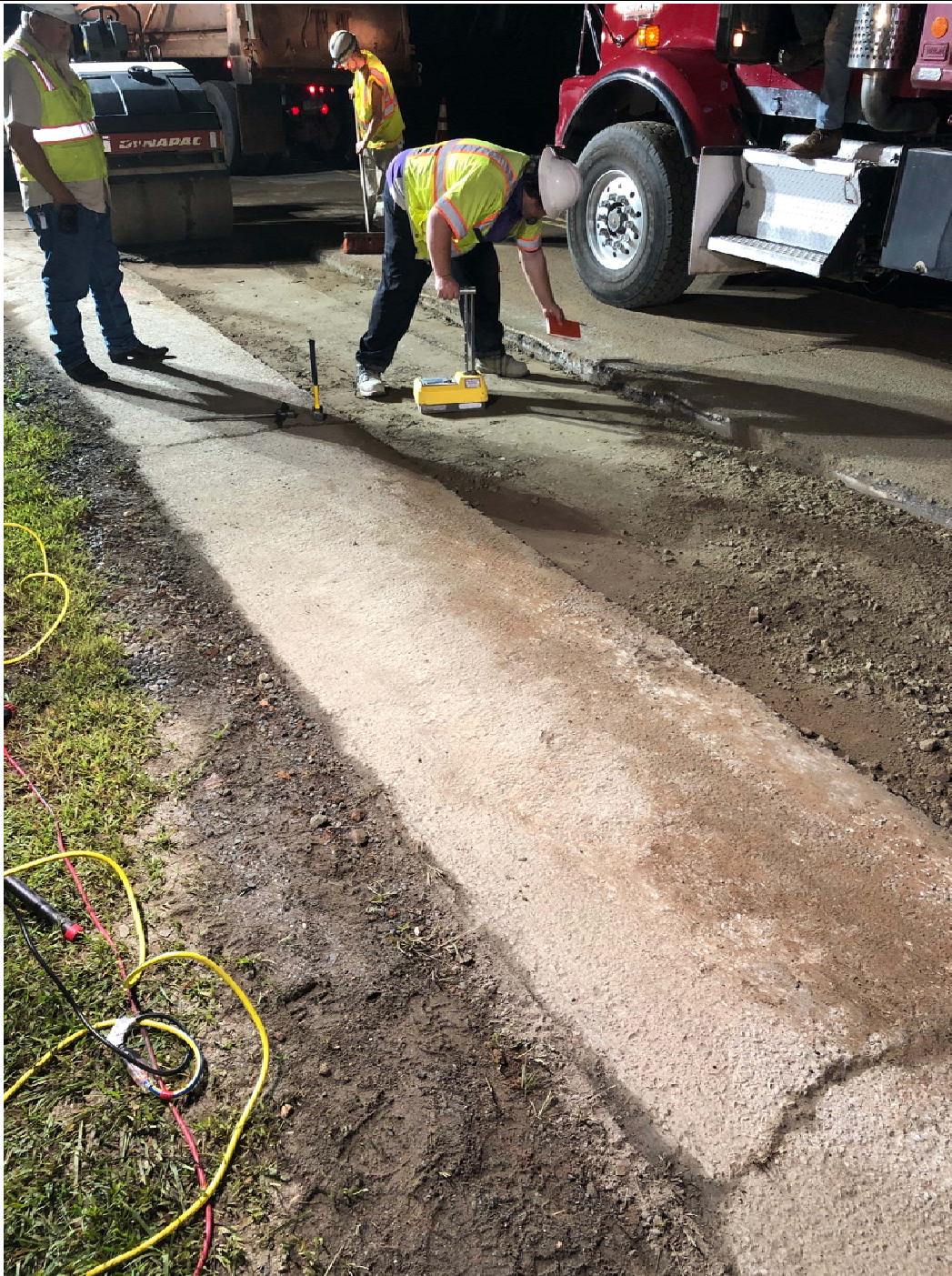
Figure 6 – Compaction testing processed stone layer
