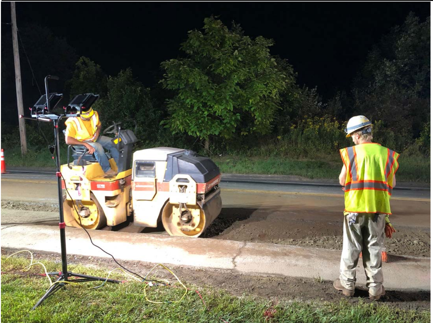
Figure 5 – Compacting processed stone
