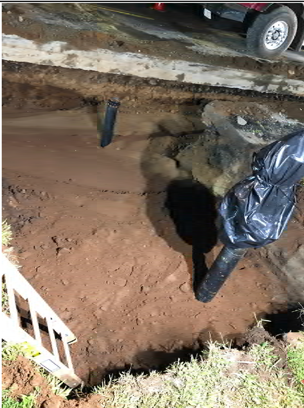
Figure 8 – Newly placed hydrant and gate valve & valve box with partially compacted 1 st fill layer
