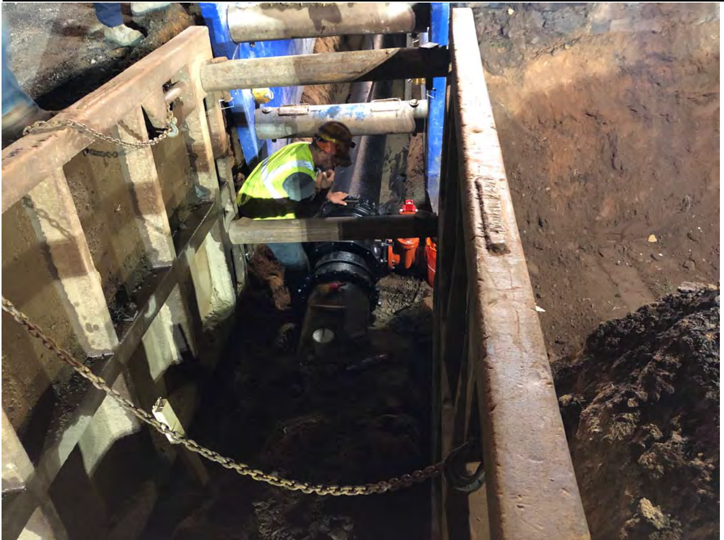
Figure 6 – hydrant tee and gate valve assembly attached to new water main
