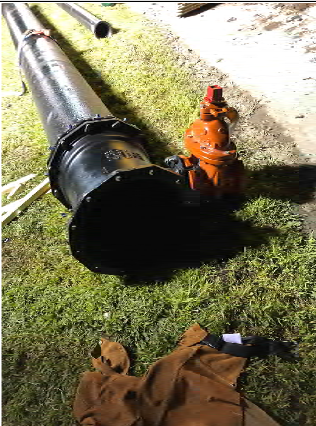
Figure 3 – Completed hydrant tee & gate valve assembly above ground
