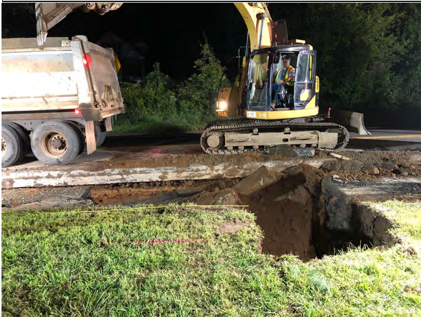
Figure 1 – Trenching for hydrant installation
