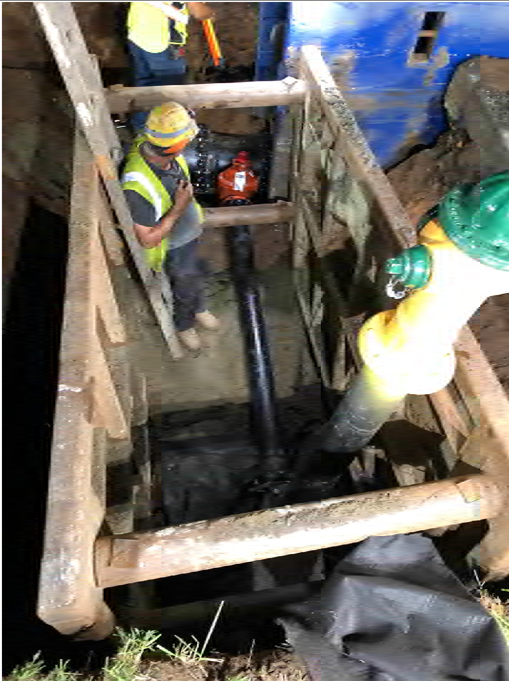
Figure 7 – Hydrant lateral attached to water main in trench
