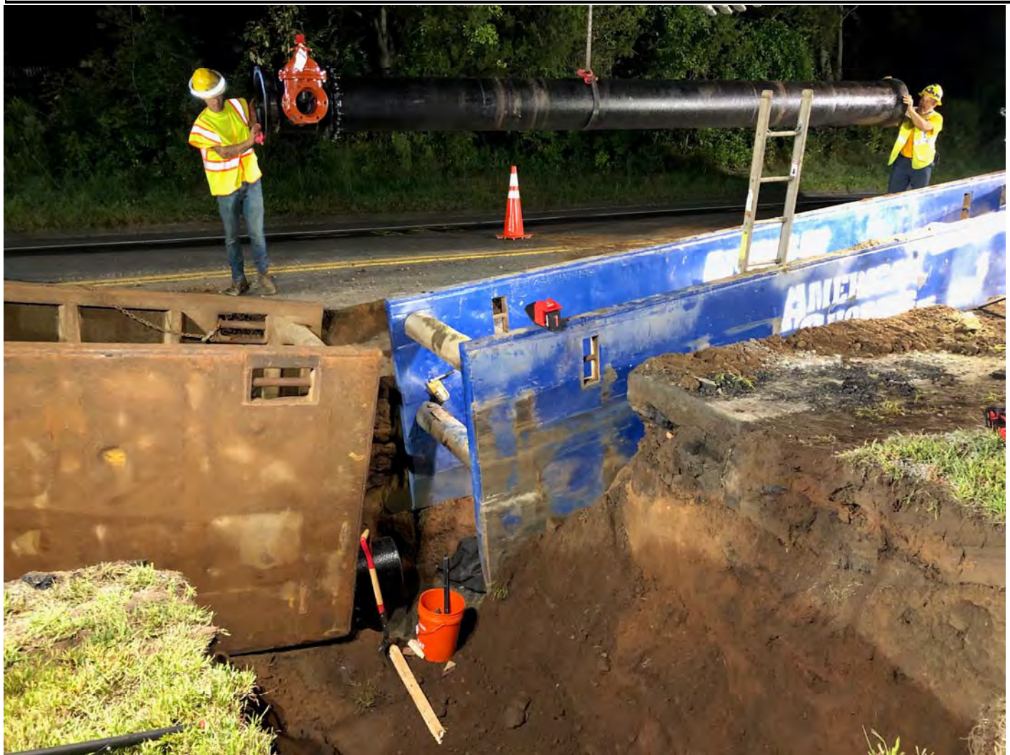
Figure 4 – Gate valve assembly and pipe length being lifted into the trench
