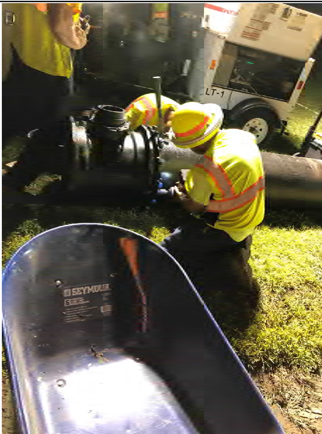
Figure 2 – Hydrant Tee being attached to water main in preparation for gate valve attachment
