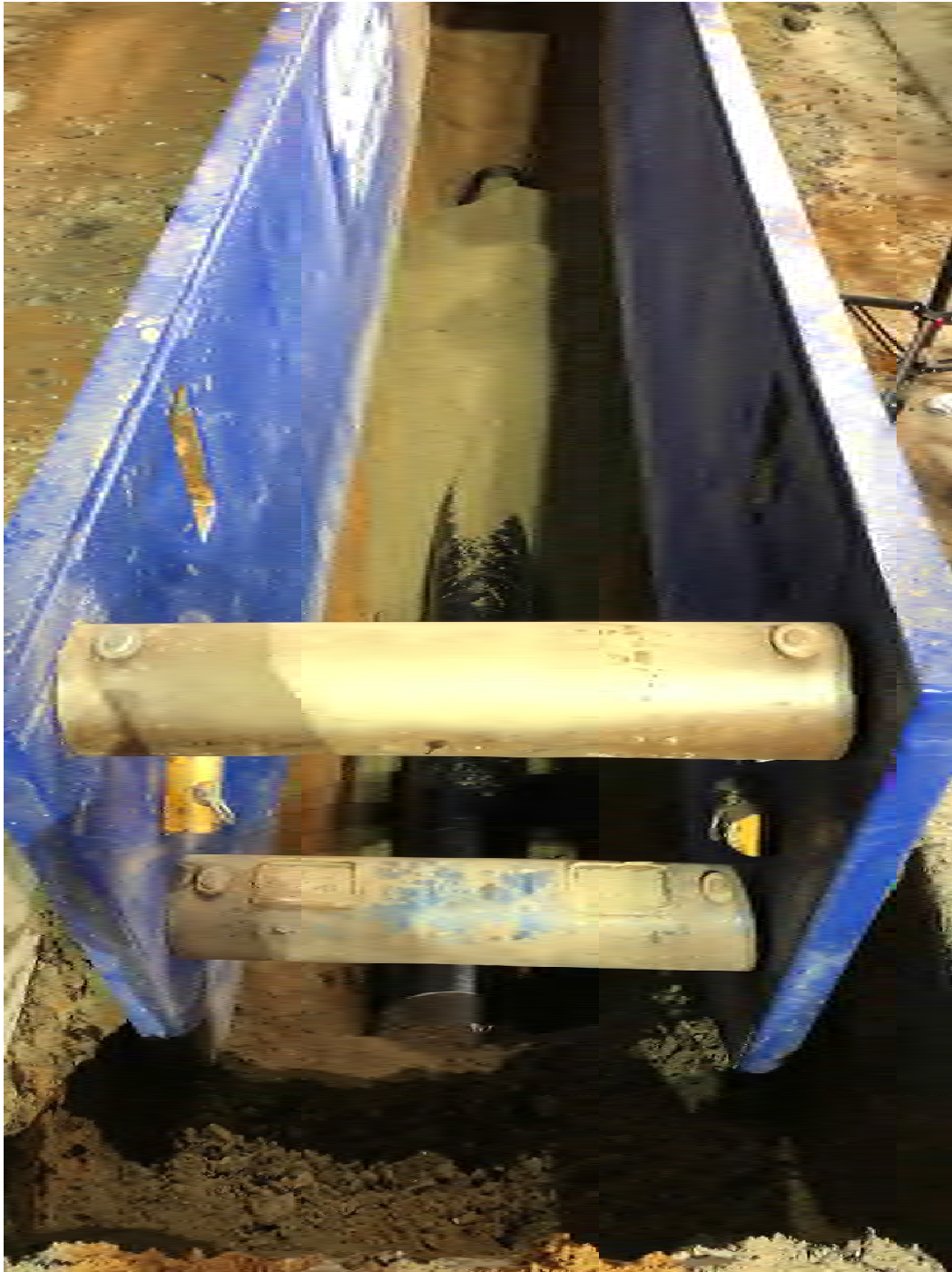
Figure 3 – Pipe Bedding being placed around newly installed pipe length, gravel wrapped in filter fabric underneath
