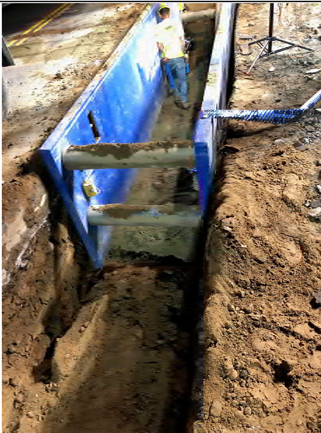
Figure 6 – Compacting first 12” backfill later above 3 rd pipe length of the night
