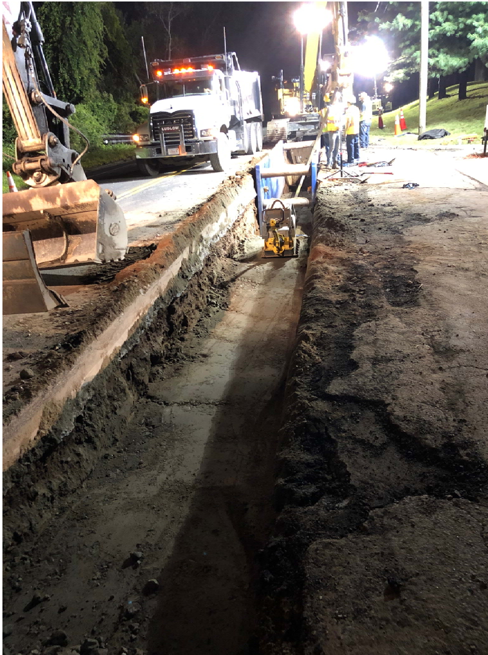
Figure 2 – Compacted top backfill layer above newly placed pipe
