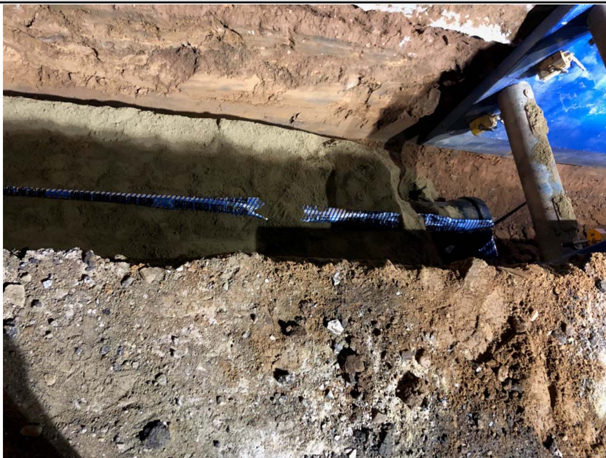
Figure 3 – Water line utility warning tape placed on 12” bedding layer above new water main
