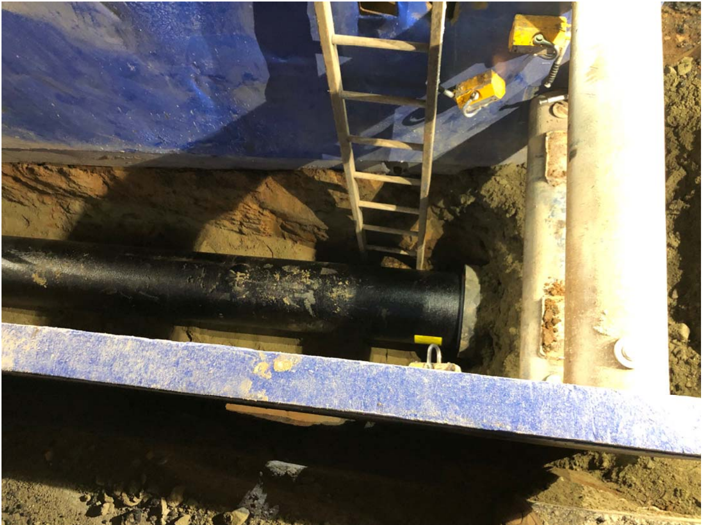
Figure 1 – New pipe section attached to end of pipe installed 9/8/19
