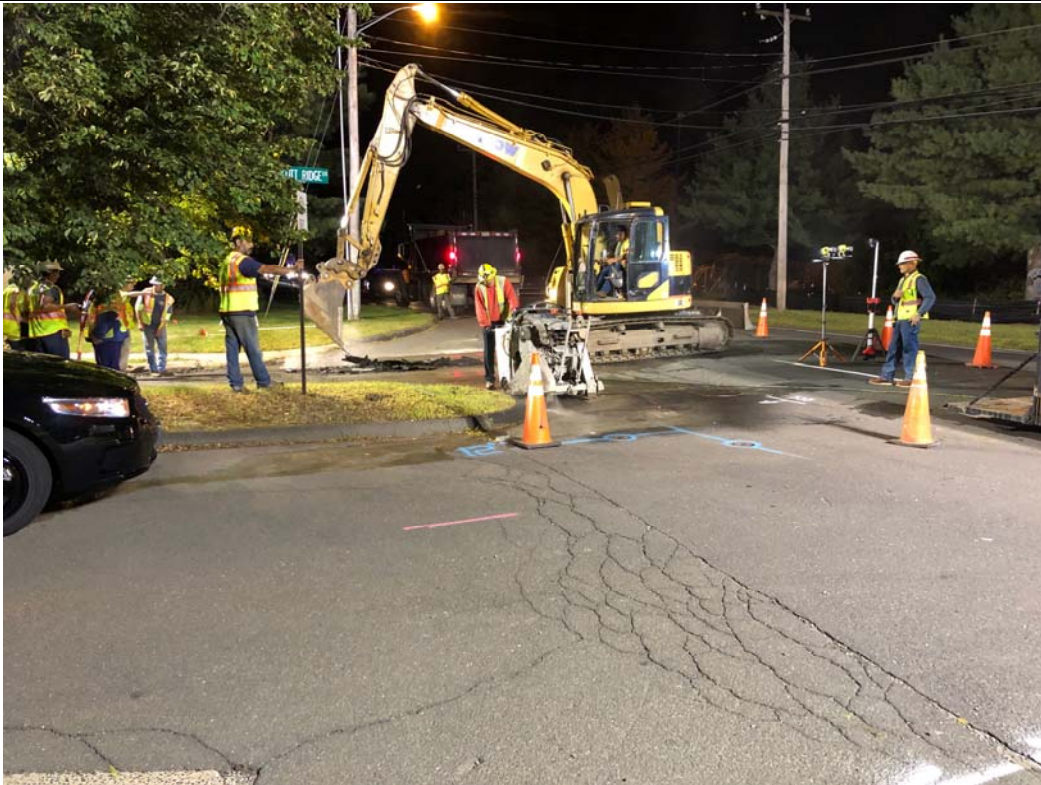
Figure 2 – Excavating Test Pit
