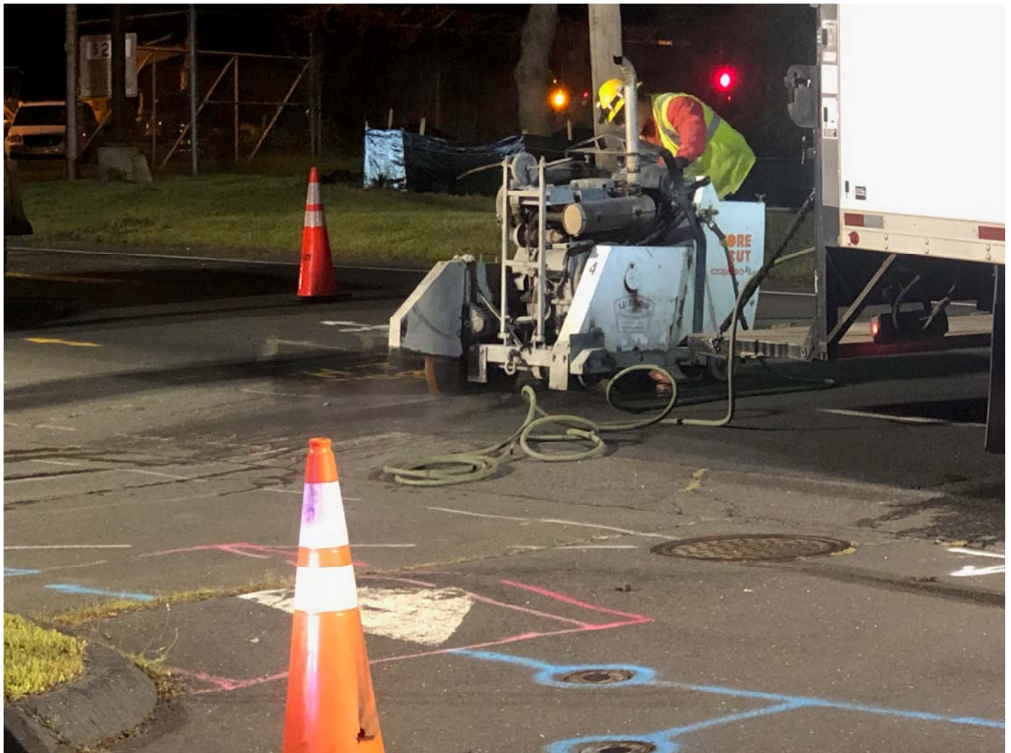
Figure 1 – Saw Cutting Pavement for Test Pit
