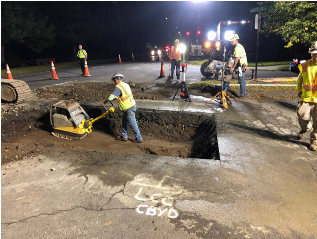
Figure 3 - Compacting Test Pit Backfill
