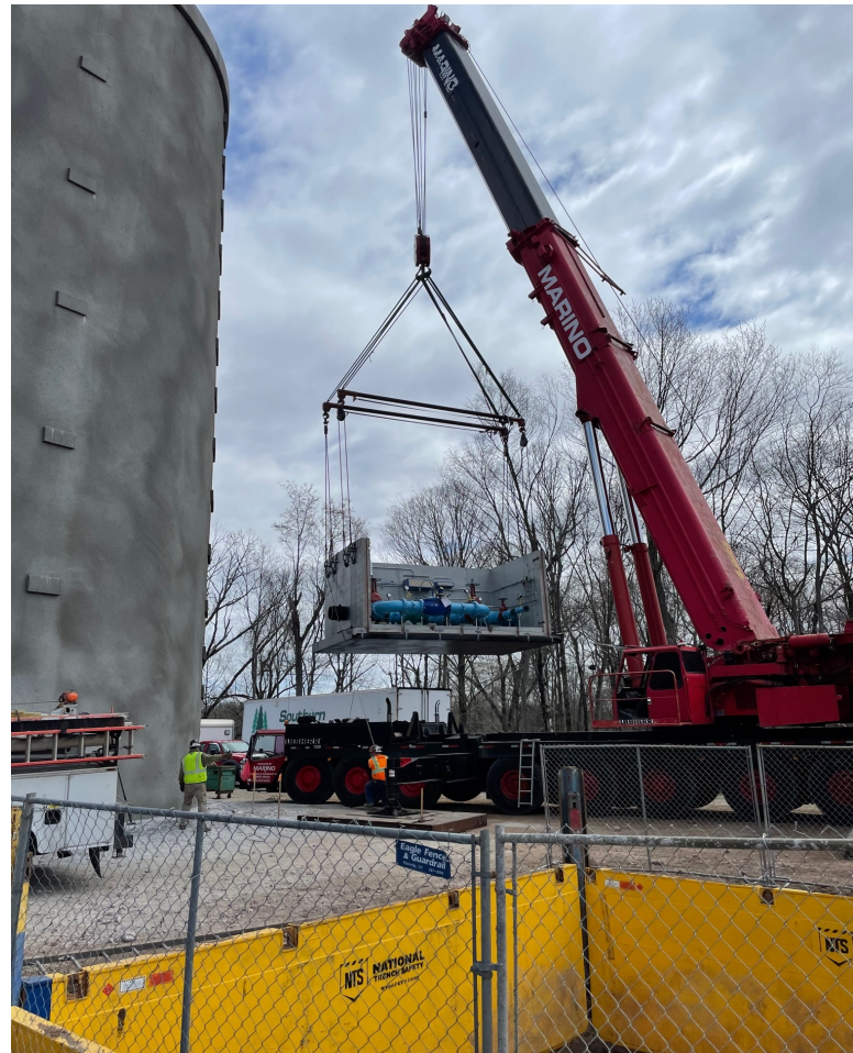
Altitude Vault Installation at Cherry Hill Water Storage Tank
