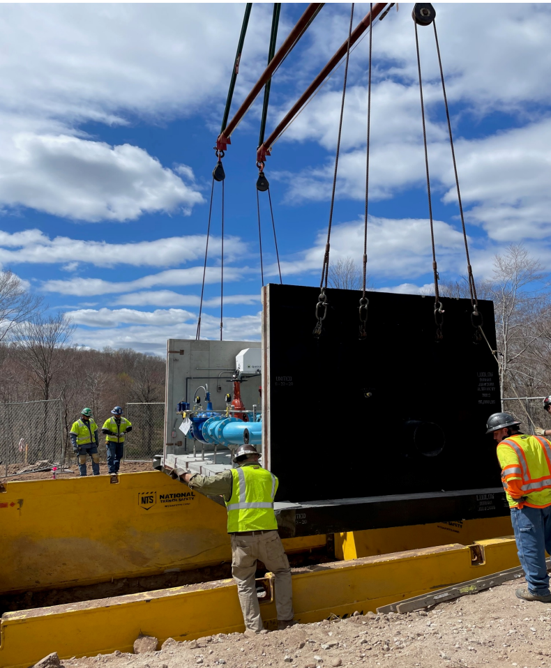
Altitude Vault Installation at Cherry Hill Water Storage Tank
