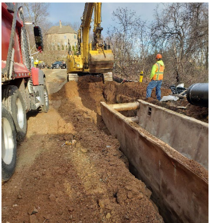
Installation of 20" DIP on Tank Access Road
