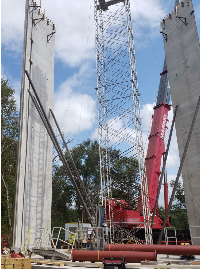
Water storage tank panels being erected
