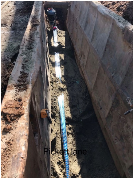
Picket Lane Water Main Installation
