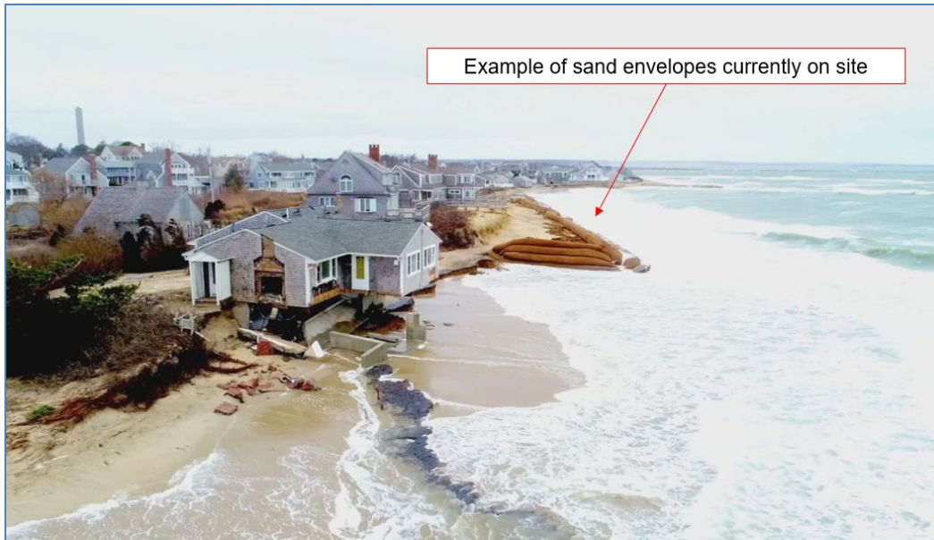
Figure 5-4: Sand envelopes (shown in Figure 5-3) following Winter Storm Riley in 2018
