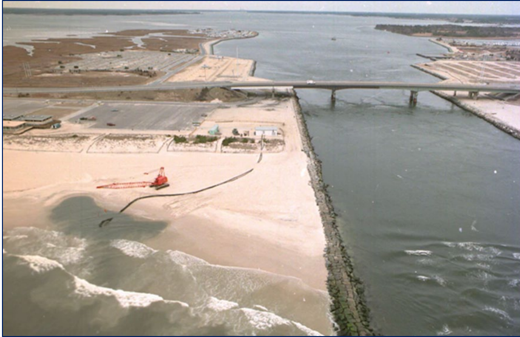
Figure 5-9: Permanent Sediment Bypass System at Indian River in Bethany Beach, Delaware
