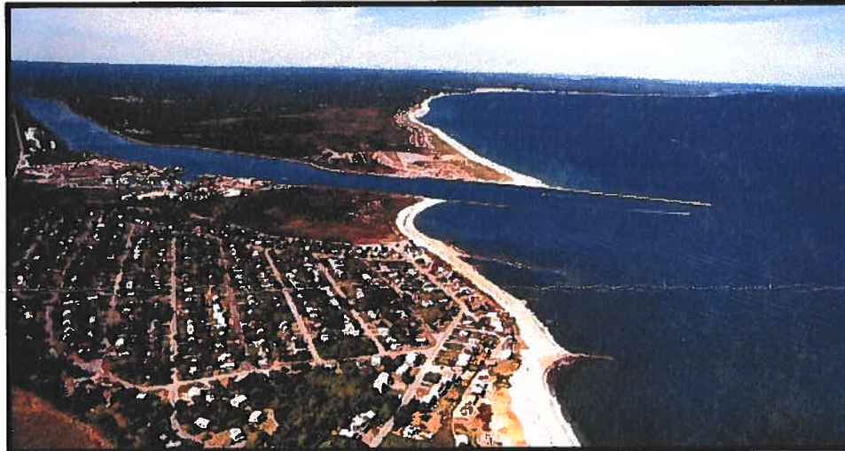
Figure 1. Eastern entrance of the Cape Cod Canal.
