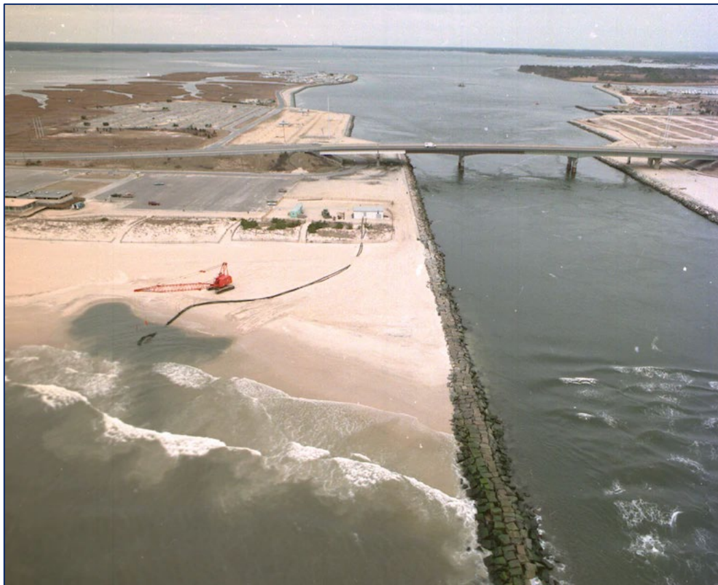
Figure E11: Example of a Sand Bypass System in place in Delaware
