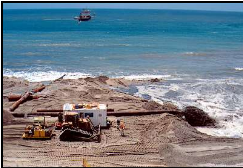
Figure 32. Beach nourishment project under construction.
