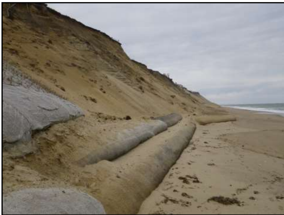
Figure 42. Example of coir envelopes exposed after storm.
