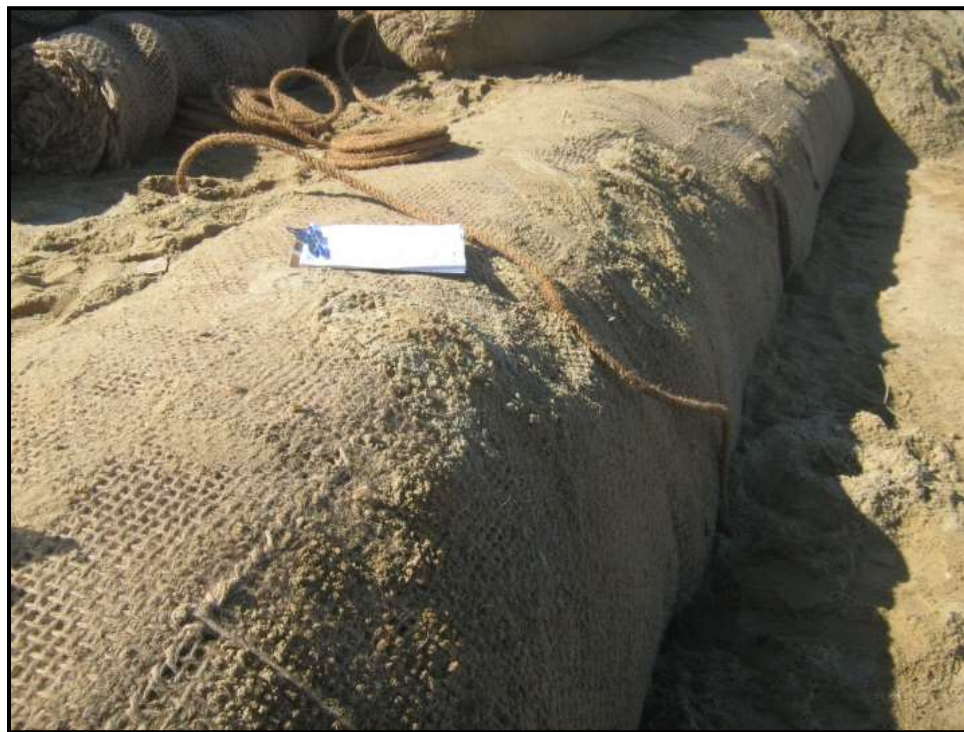
Figure 41. Biodegradable coir sand filled bag during construction.
