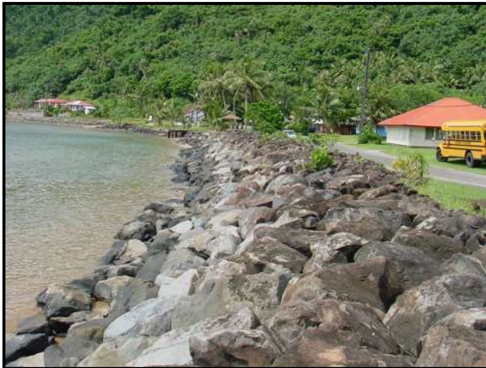
Figure 56. Example of a typical revetment.
