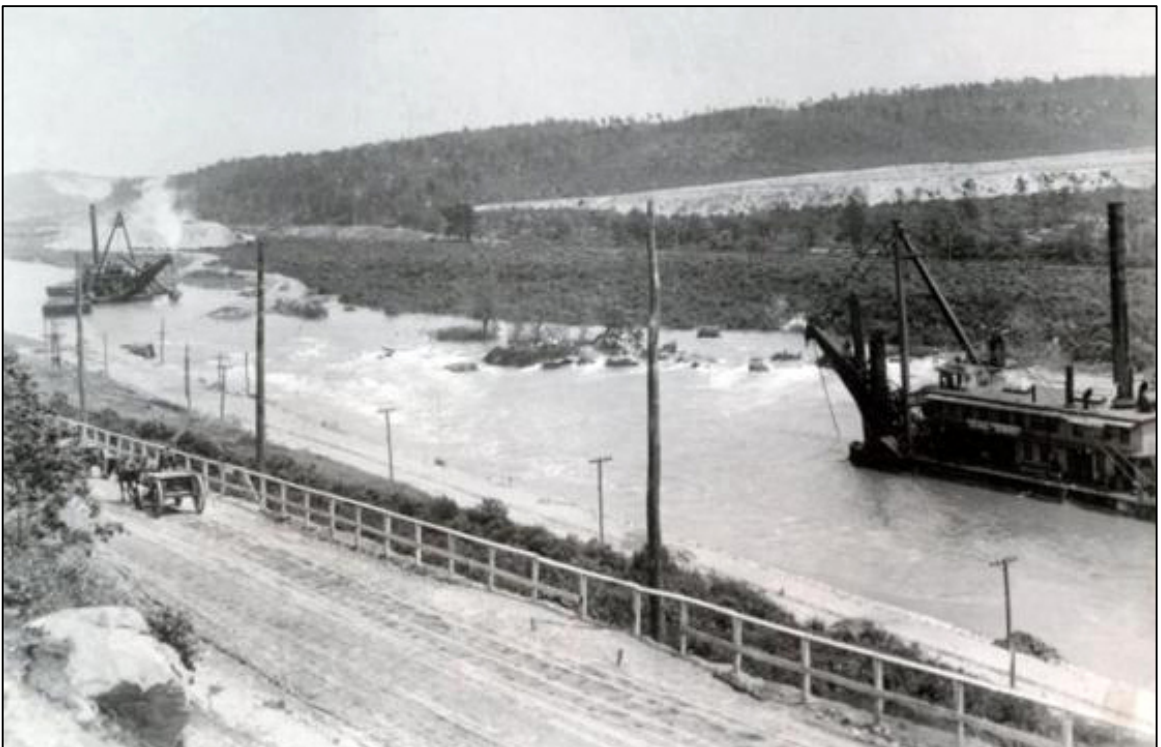
Image 10. View of excavation of the Monument River, with two dredges working toward each other, ca. 1912 (from Town of Bourne website historical photos).
