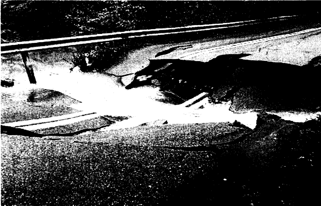
Figure 2: Road washout in Lincoln, RI.
