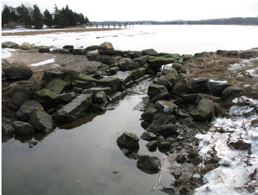
Abandoned cart path fill across upper Apponagansett Bay blocks intertidal channel and restricts tidal flow. Dartmouth, Massachusetts
