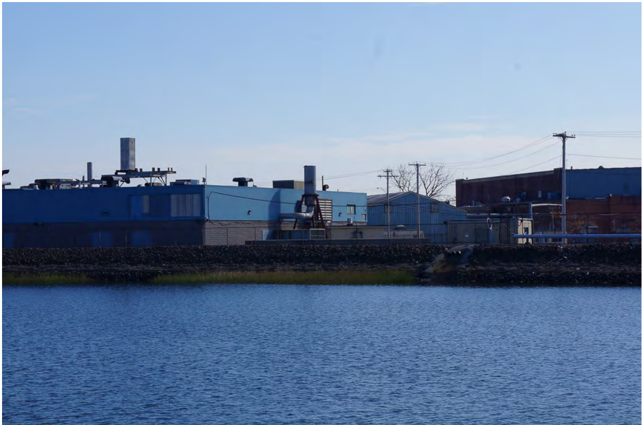
Photo 11. Mid - Causeway looking southeast across east tide flat to eastern end of dike and revetment, mid-tide. October 6, 2017.
