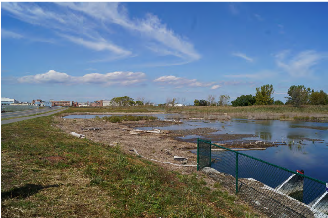
Photo 2. East of Outfall 008 Drainage Ditch confluence with tidal lagoon, looking northwest. October 6, 2017.
