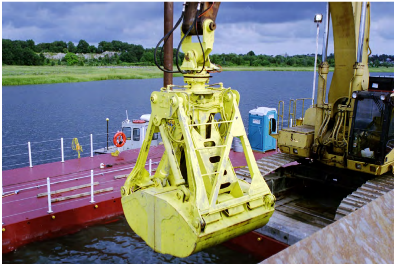
Figure 6. Alternative 3 - Precision Excavator - Hydraulic Transport Dredge with 4.6 cy (3.5 m 3 ) Horizontal Profile Grab Level-Cut Environmental Clamshell Bucket, New Bedford, MA, 2000.
