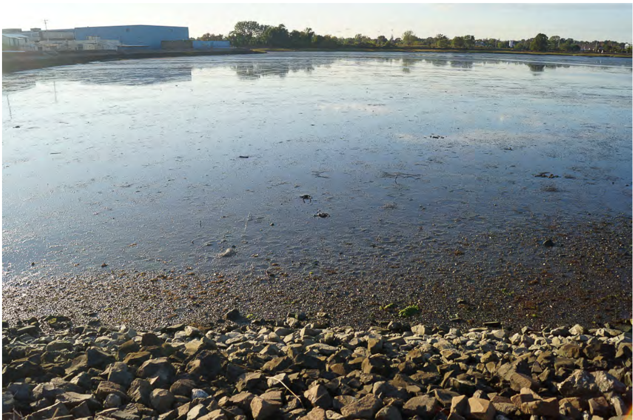
Photo 12. South Causeway on rock revetment looking west across west tide flat, near low-tide. October 6, 2017.
