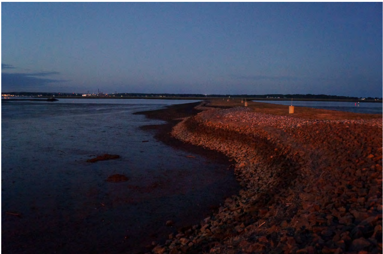
Photo 20. South Causeway looking north. October 6, 2017.
