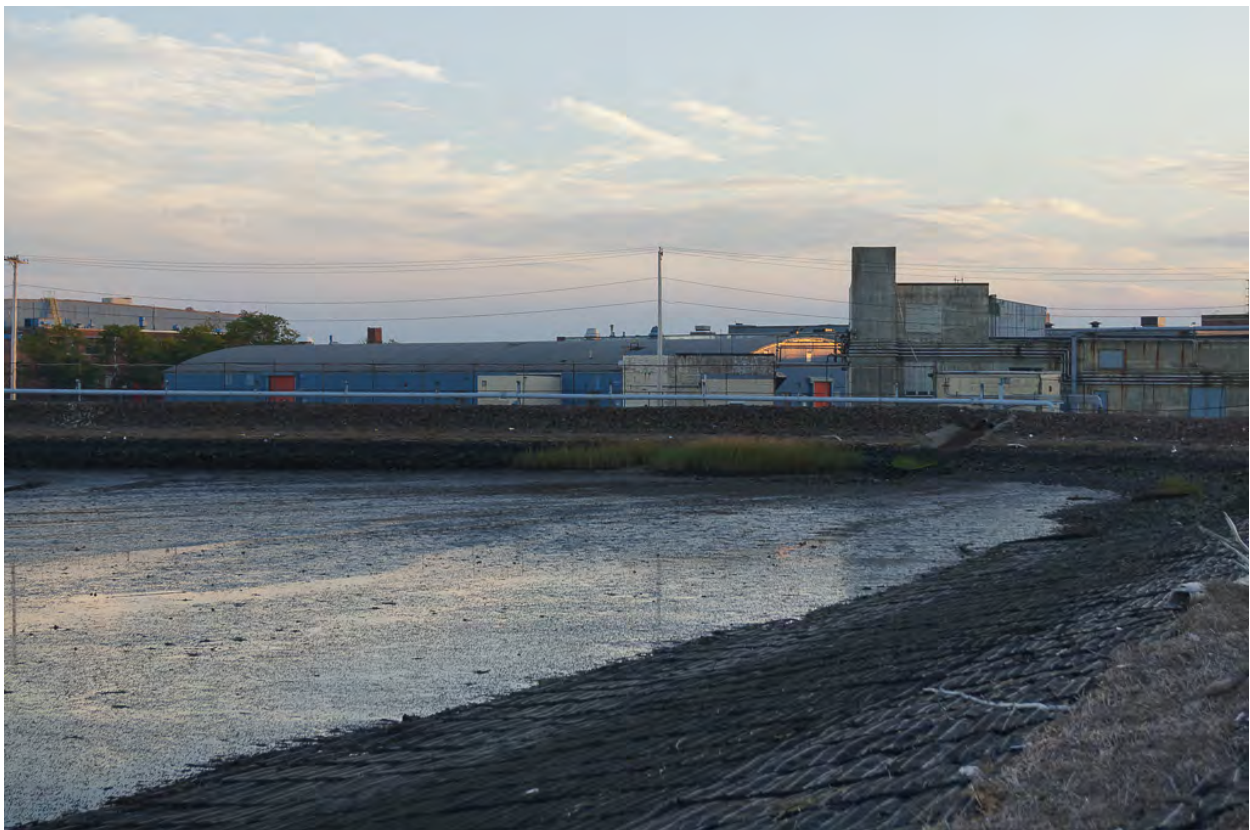
Photo 14. Mid - Causeway looking southeast across east tide flat, near low-tide. October 6, 2017.
