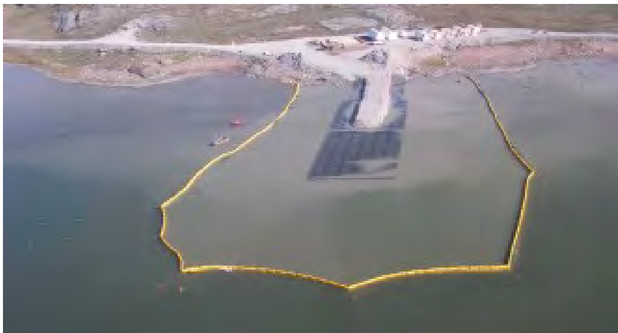
Figure 14. Engineering Control – Turbidity Barrier. Source: Layfield
