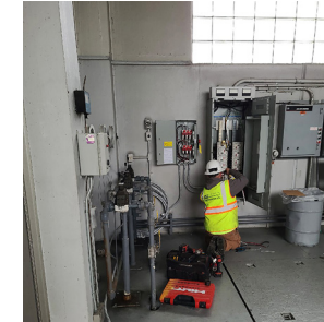
Conduit and wiring replacement, North Springfield Lake, North Springfield, Vermont.
