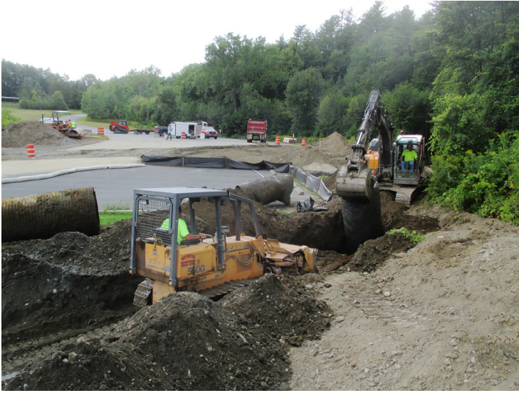
Culvert replacement, North Hartland Lake, North Hartland, Vermont.
