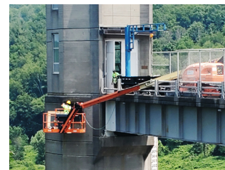
Replacement of vent grate, Thomaston Dam, Thomaston, Connecticut.
