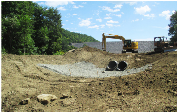
Culvert replacement, North Hartland Lake, North Hartland, Vermont.
