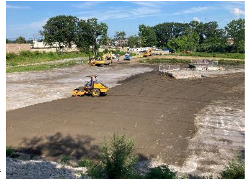
Material placement work Raymark Superfund site, Stratford, Connecticut
