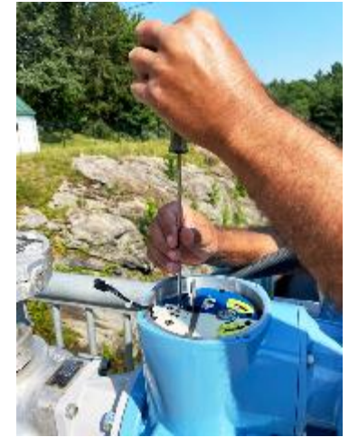
Contractor adjusting the gate operator upper and lower limits at West Hill Dam, Uxbridge, Massachusetts
