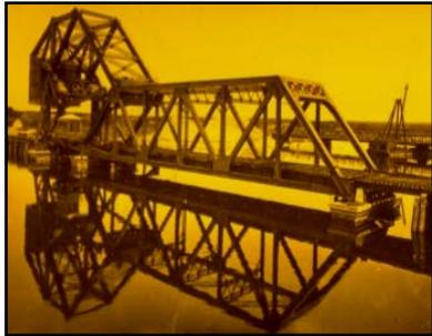
The 160-foot span pivoted on the north side of the Canal utilizing a single counterweight. The bridge in the raised position had an opening of 140 feet for vessels passing through. Two tracks crossed the bridge, one heading towards Provincetown and the other towards Woods Hole.
