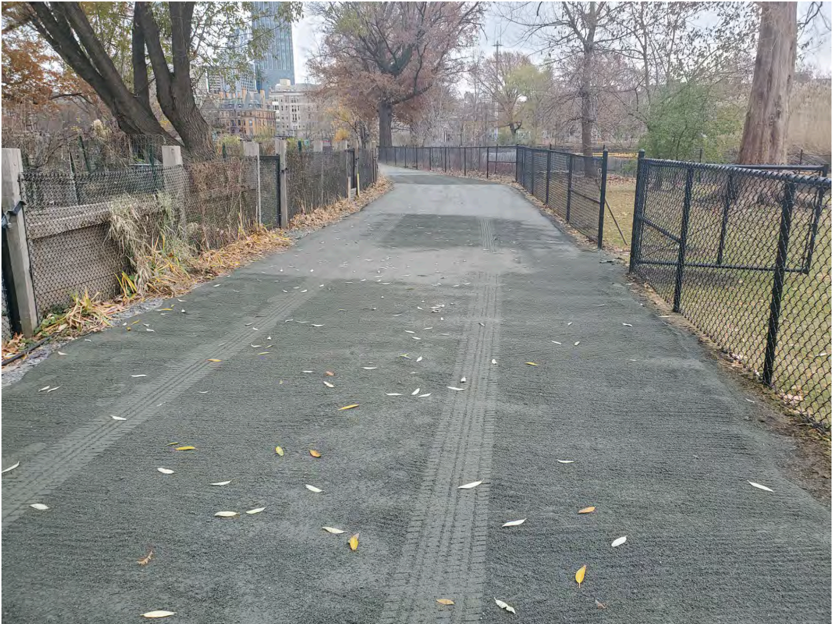
Work Area #11 – Victory Gardens Area – stonedust pathway restored.
