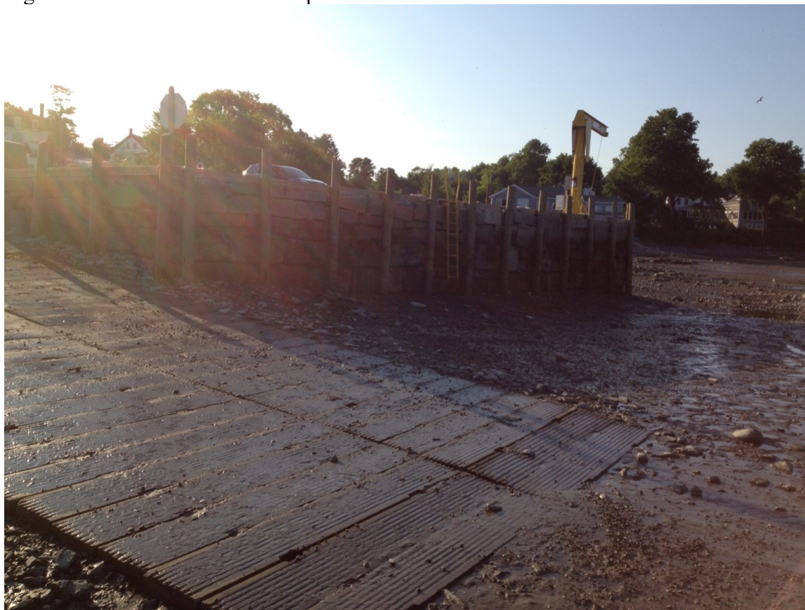
Figure 2. Bulkhead and boat ramp of the Blue Hill Harbor town wharf.
