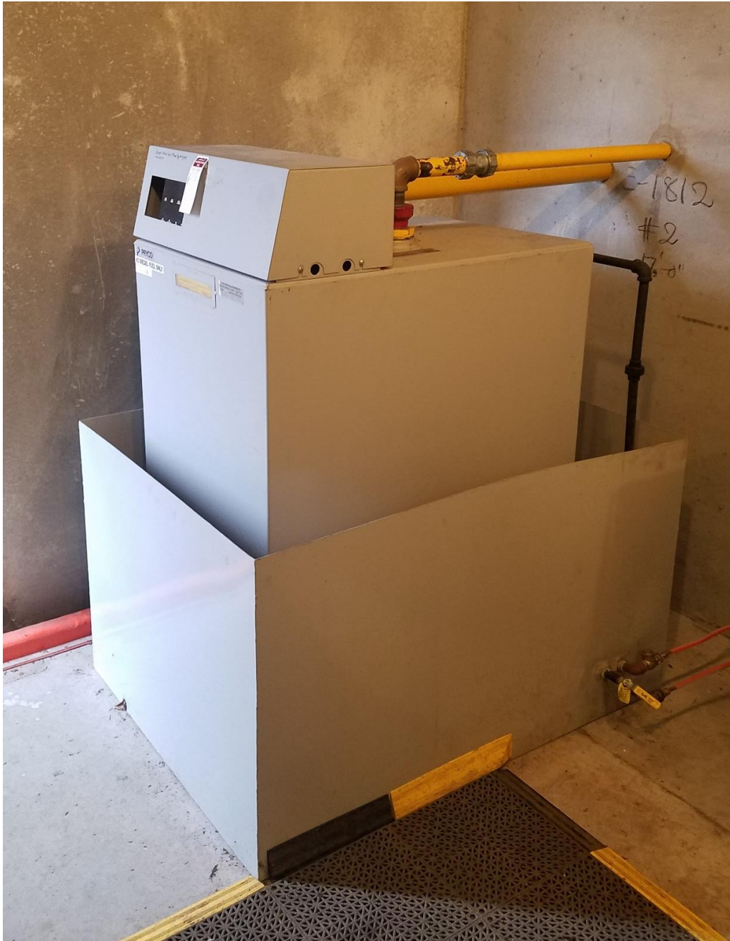
Photo 1: View of tank and containment basin (East Brimfield Lake)
