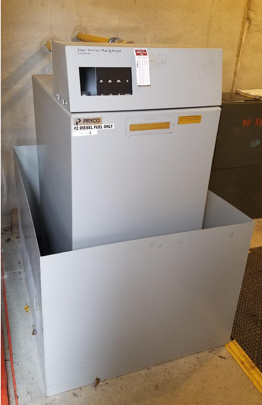
Photo 2: View of tank and containment basin (East Brimfield Lake)
