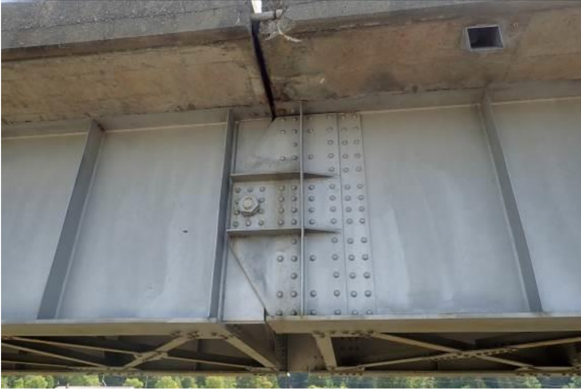
Informational Photo 2: Typical Girder Pin on North Springfield Lake Service Bridge
