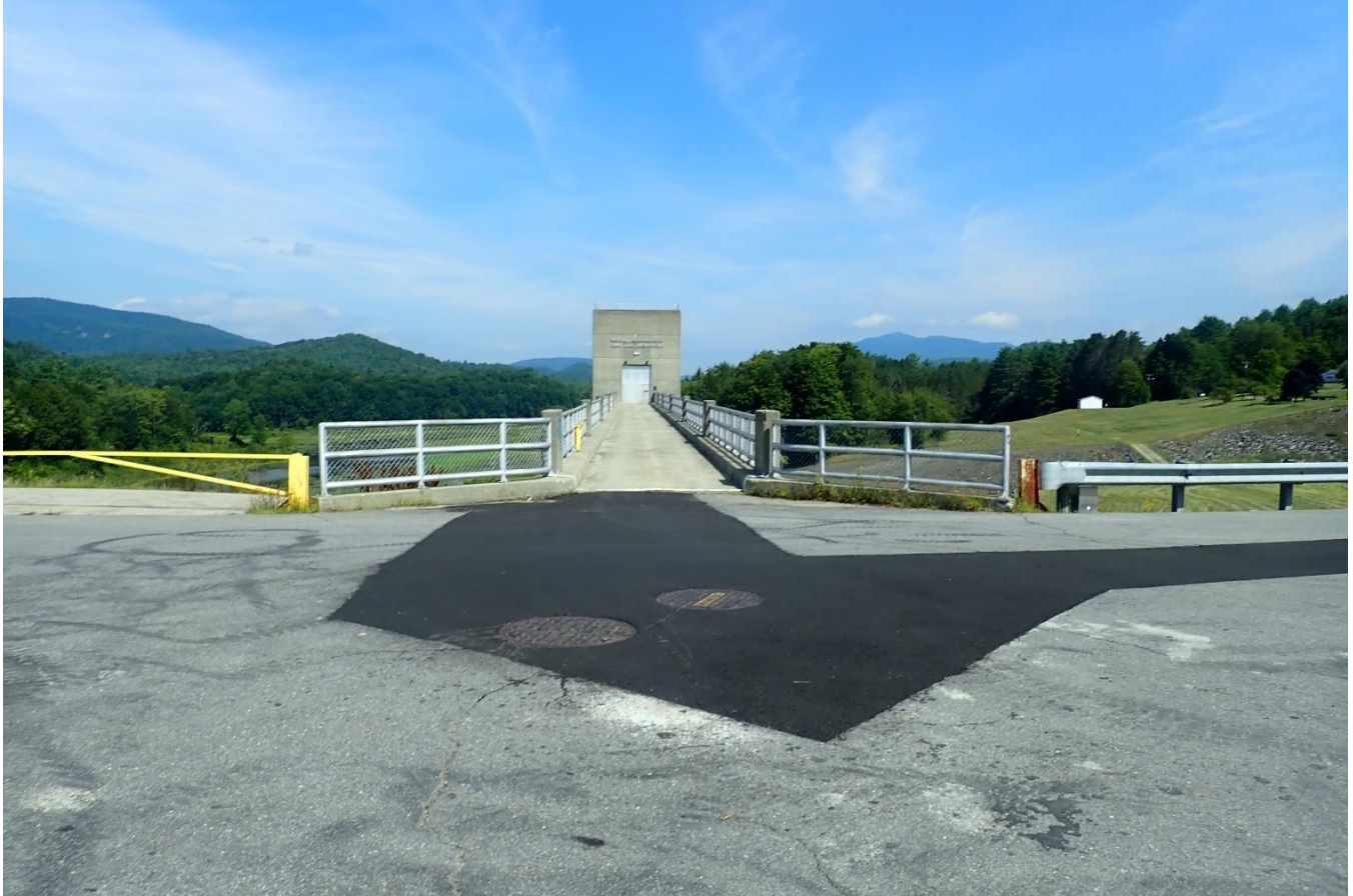
Informational Photo 3: North Springfield Lake Service Bridge Approach
