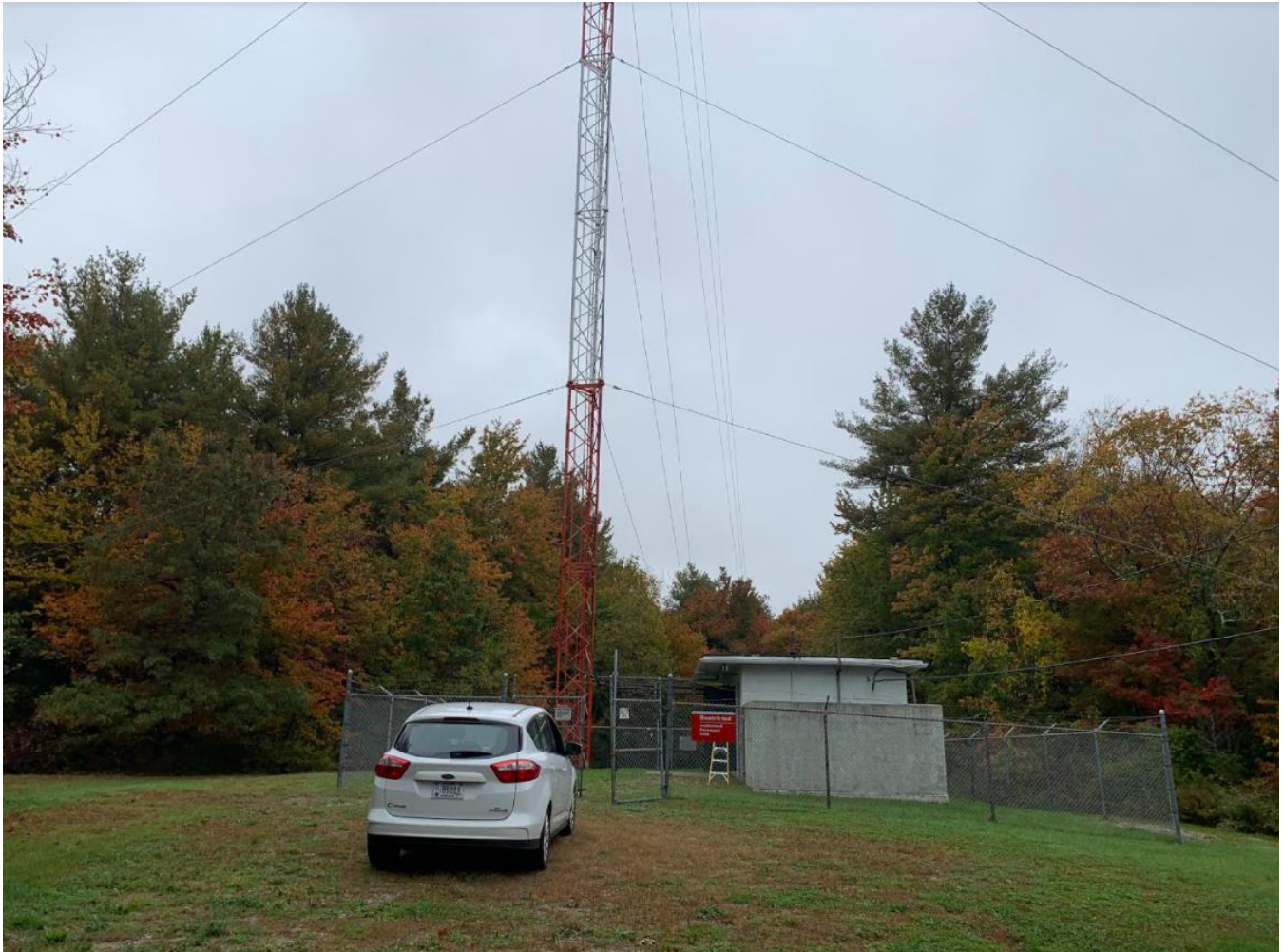
Exhibit A: Front view of Goshen Relay Radio Tower and Station
