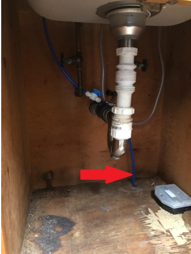
Exhibit L: Existing kitchen sink with water filter faucet (circled in red) to be saved and re-installed in a similar position on the new sink. Also shown is the supply line from the filter system to the filter faucet (red arrow)
