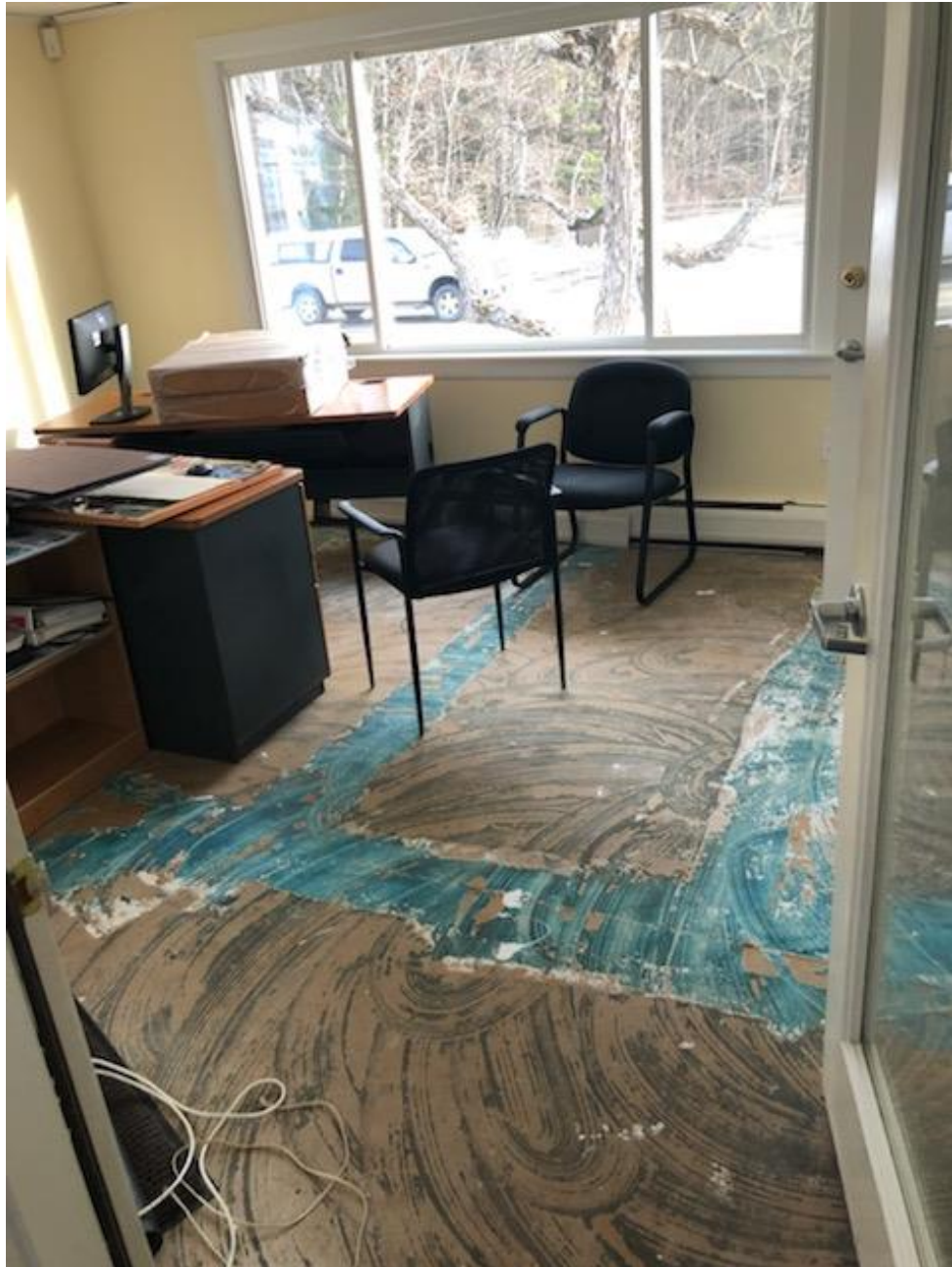
Condition of Subflooring and trim in Manager's Office
