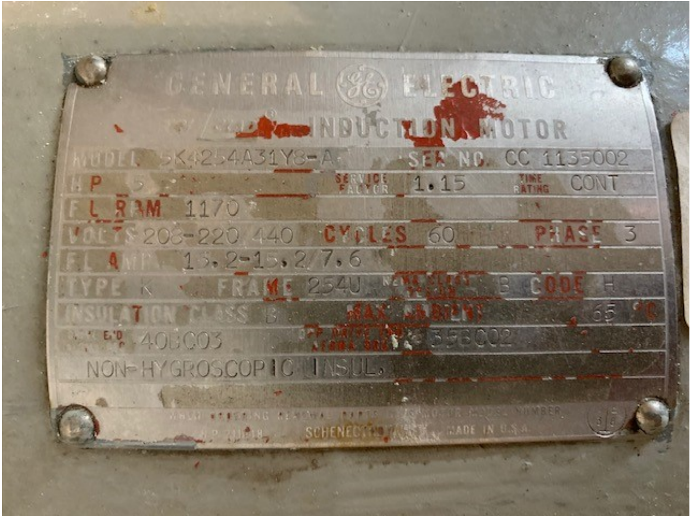
Informational Photo Number 2: General Electric Tri-Clad® Induction Motor #1 Data Plate
