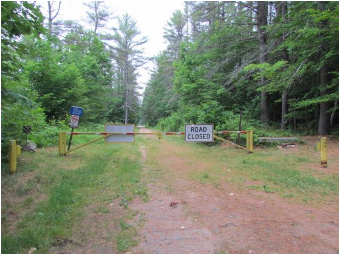
Figure 3: Typical view of 3" steel double swinging arm gate to be painted, with locking posts pictured
