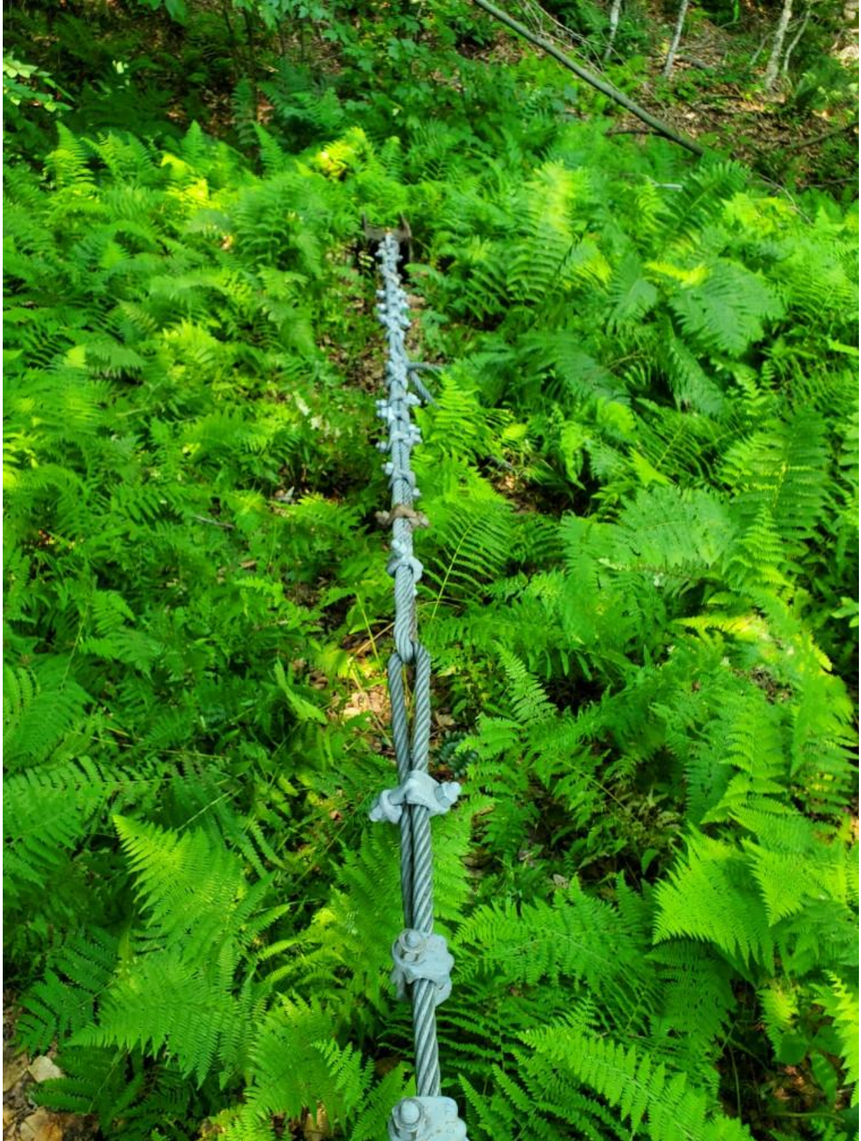
Informational Photos 4: West Shore log boom wire connection
