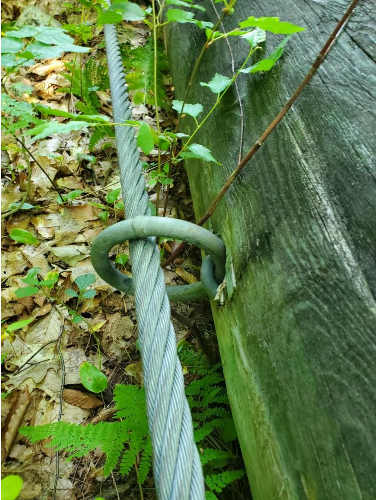
Informational Photos 5: Log boom ring connected at log
