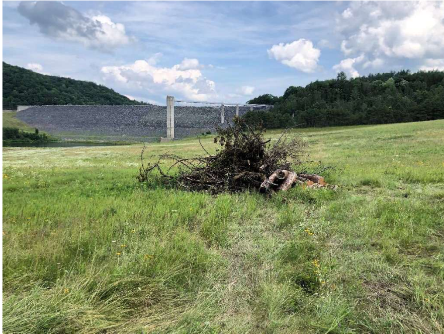
Photo 3: River Debris Pile #2
