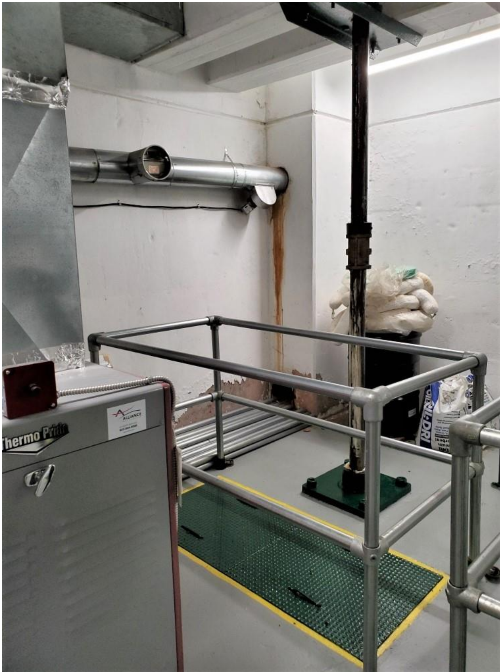
Exhibit D – Heater Room Floor chimney and furnace
