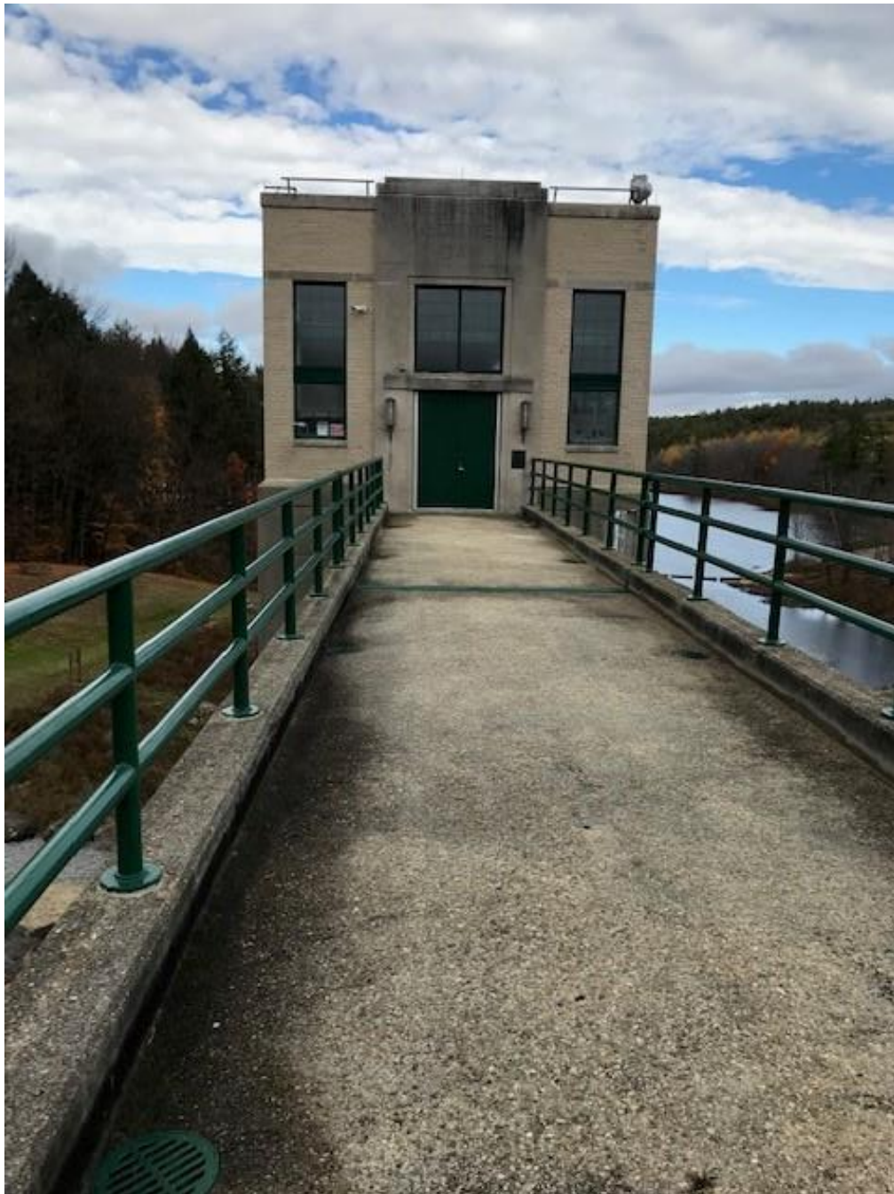
Exhibit B - Service Bridge leading to Operating Floor
