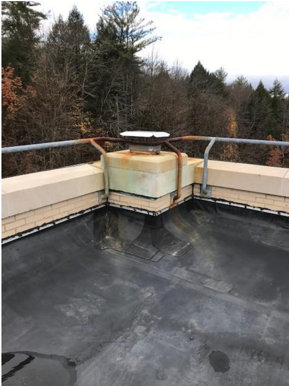
Exhibit F – Chimney location on rooftop
