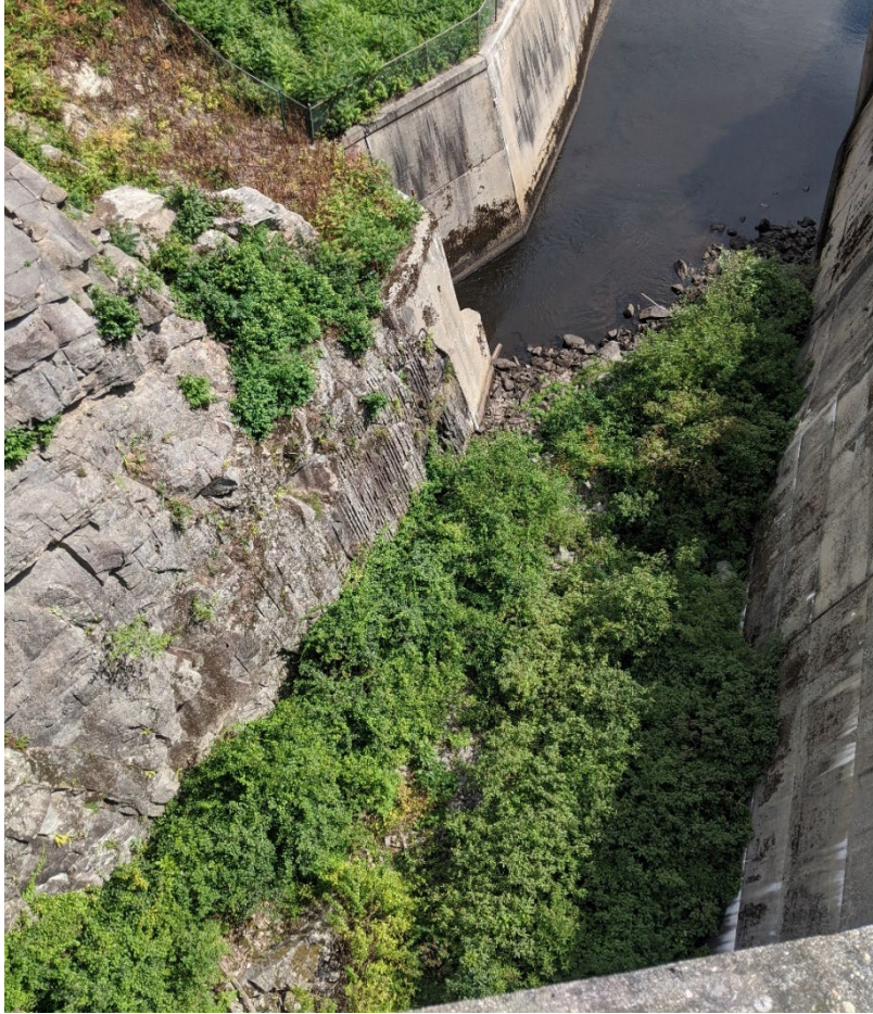
Photo 5: Vegetation conditions on east side of spillway ledge slope, southern portion. Vegetation conditions on spillway floor, southern portion.
