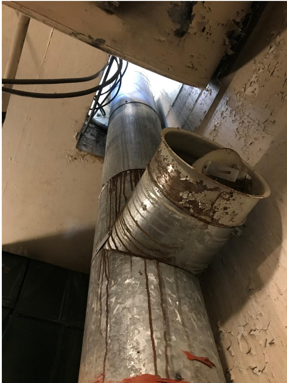
Informational Photo 3: Duct work to be replaced
