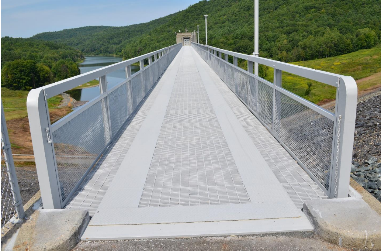
Informational Photo 5: Access to gatehouse via 5 ton limit bridge
