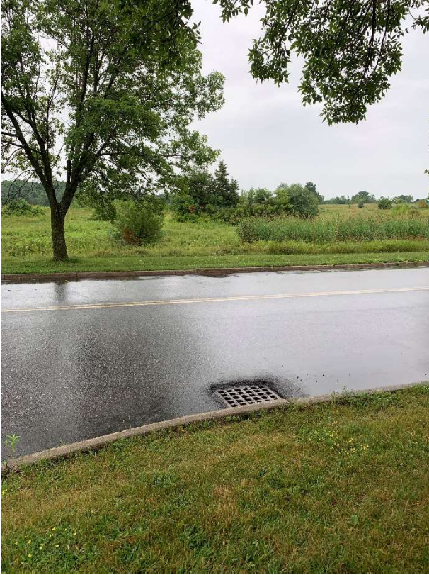
Photo taken 4 August 2020. Facing south across Swift Street looking at catch basin and Wetland B.
