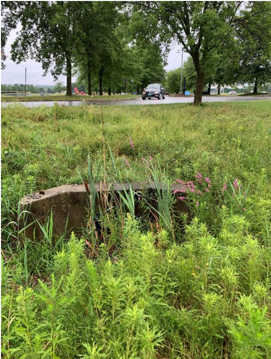
Photo taken 4 August 2020. Facing north towards 18" culvert beneath Swift Street from Wetland B.
