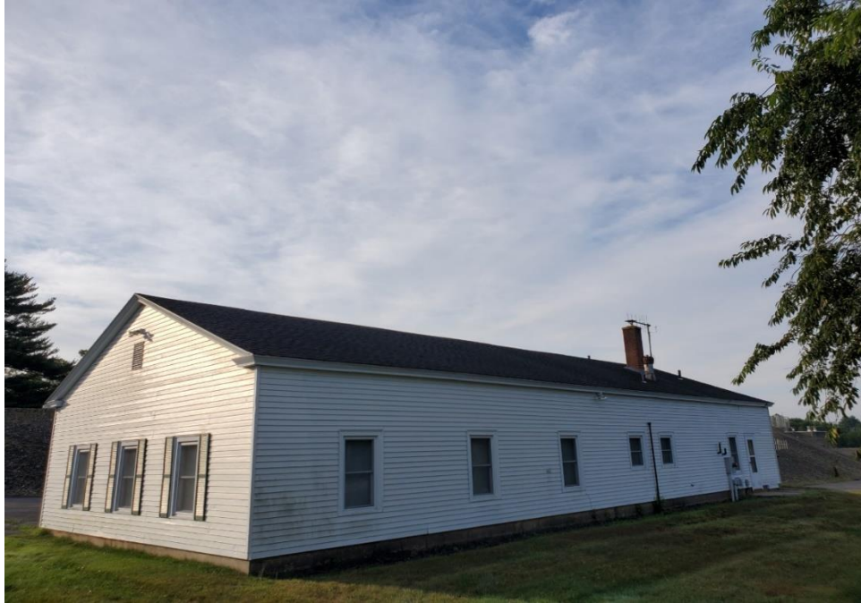
Photo 5: Rear/Side view of Utility Building
