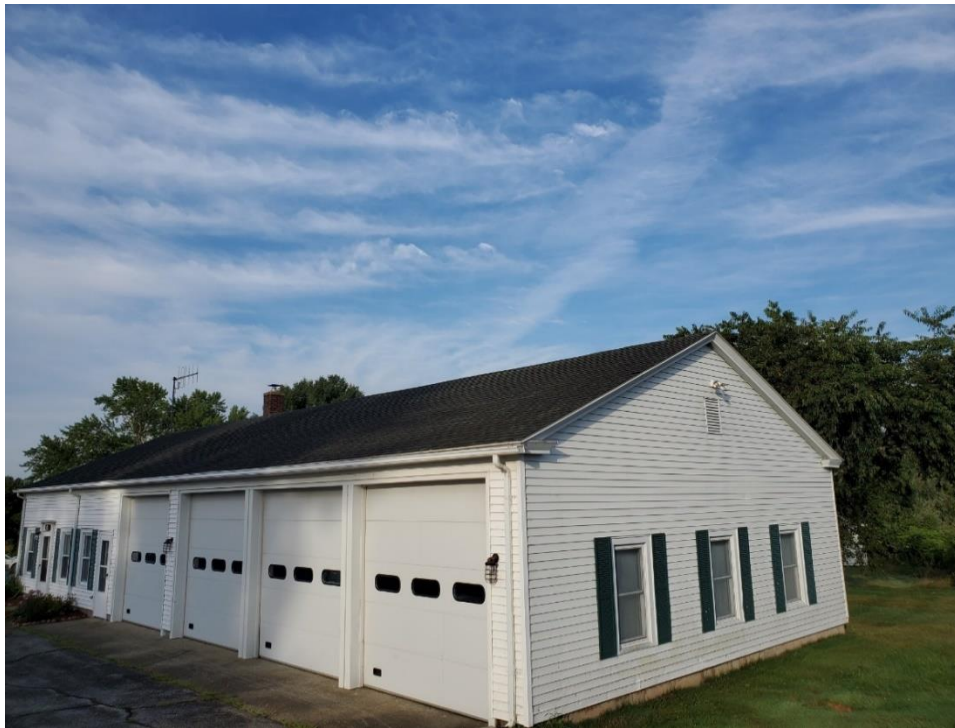
Photo 4: Side view of Utility Building
