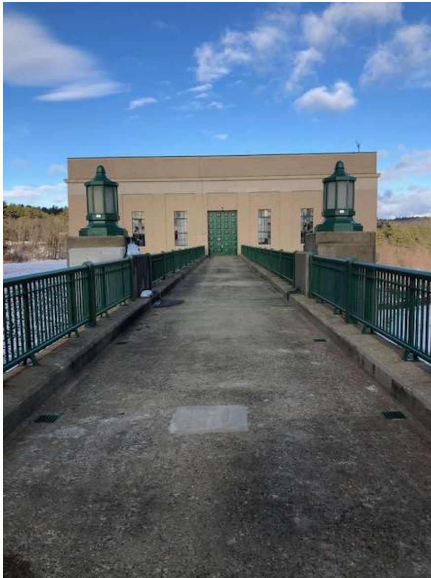
Exhibit A: Franklin Falls Dam Gatehouse Service Bridge.
