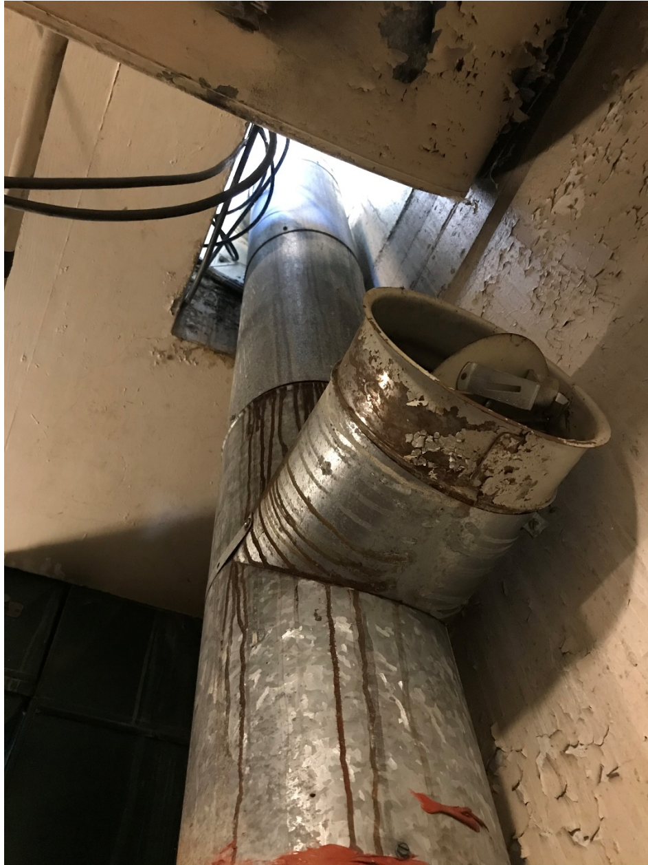
Informational Photo 3: Duct work to be replaced
