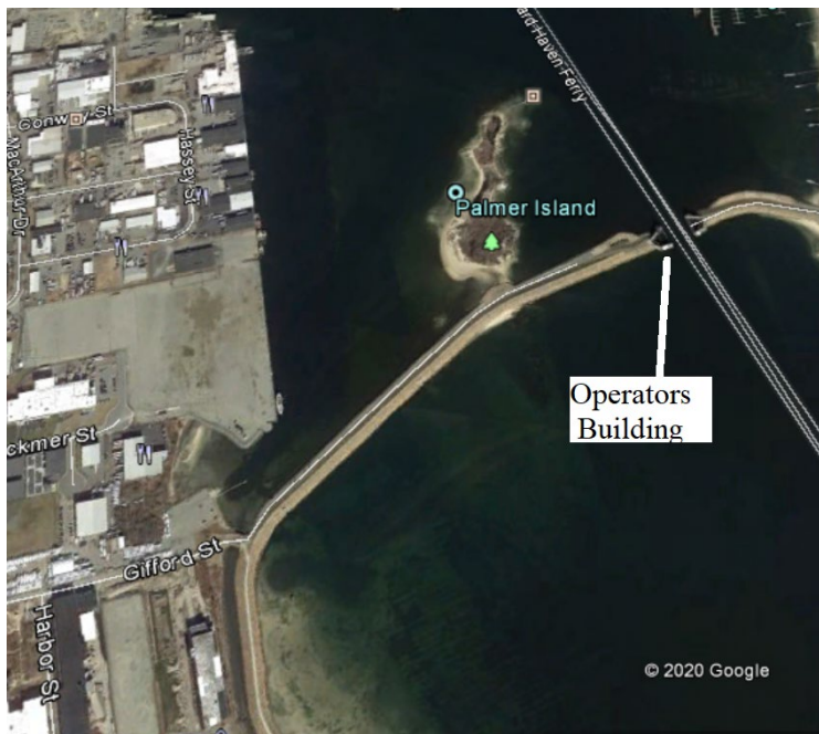
Figure 2 shows general location of Operating House #1 with access via road on dike.
