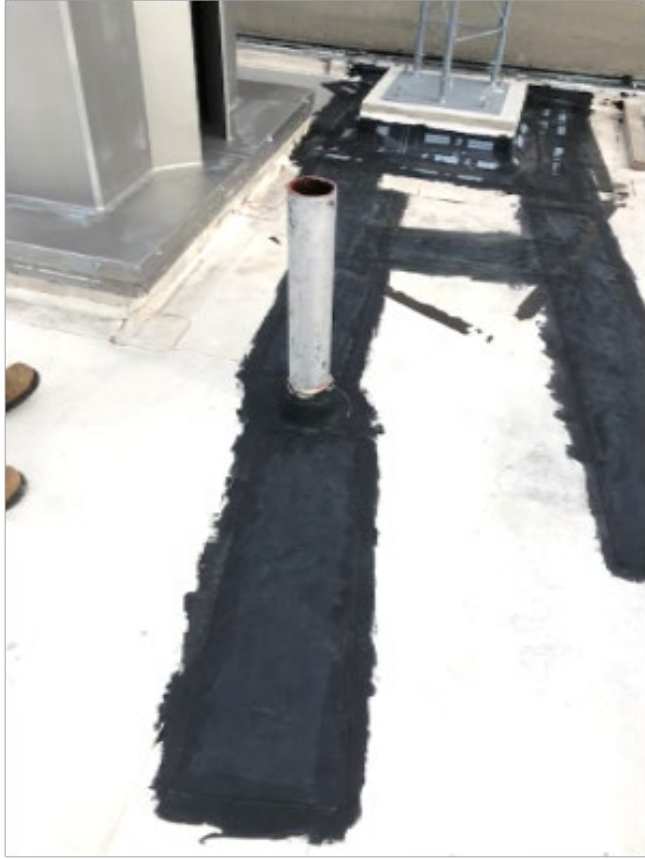
Photo 5: Shows temporary patch materials with existing PVC membrane, looking east.
