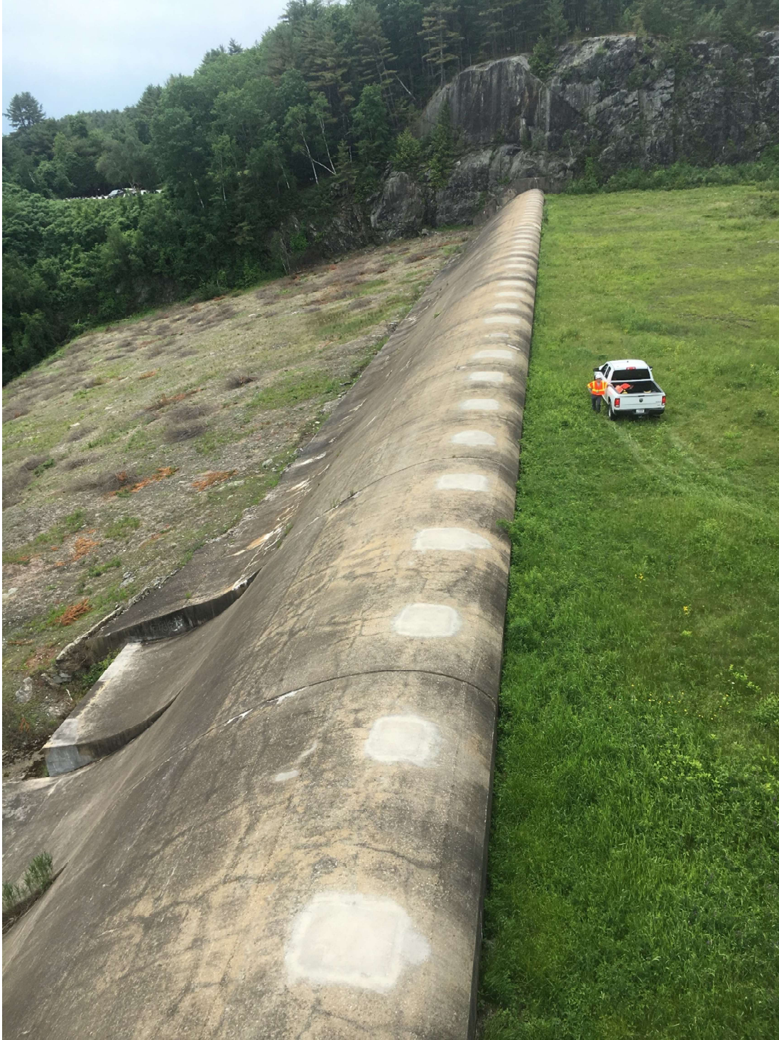
Reference View of Spillway Weir at the Franklin Falls Dam
