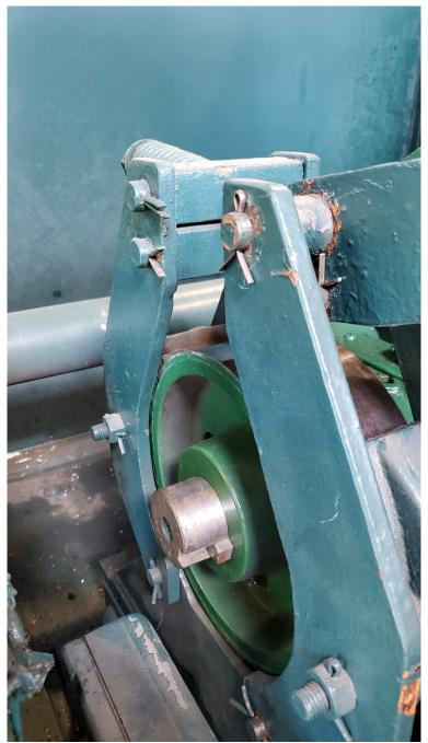
**Photo 8:** Side view of brake and rotor on gate hoist 1. Showing glazing on face of rotor and wear on the size of the rotor due to movement in the armature shaft
