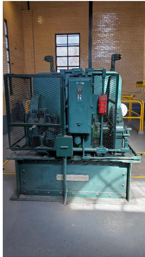
**Photo 1 & 2: Gate Hoists 1 and 2 as seen from the front**
