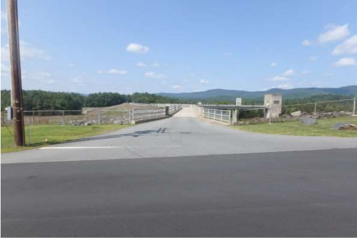
Photo 17: North Springfield Dam Spillway Bridge – Plan View
