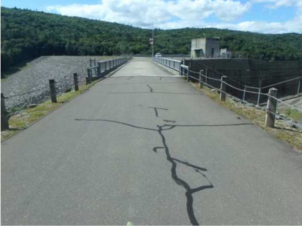
Photo 7: Littleville Lake Spillway Bridge – Plan View
