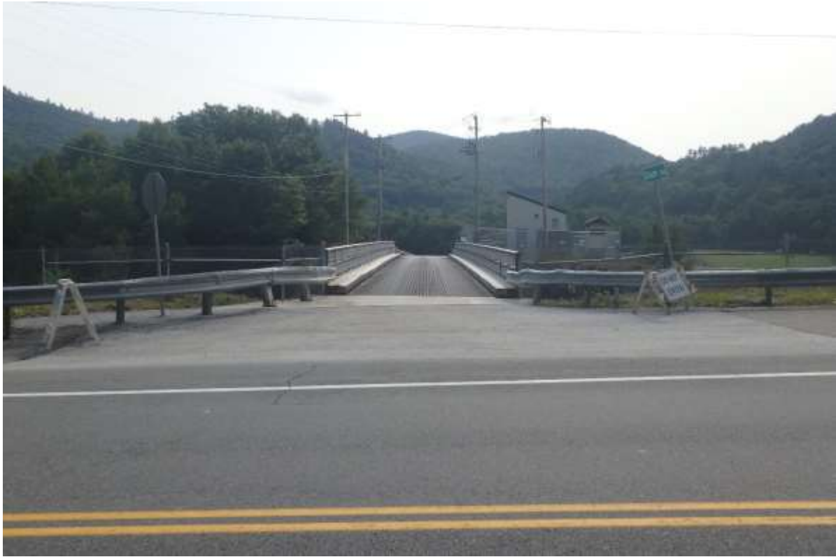
Photo 19: Townsend Lake Spillway Bridge – Plan View
