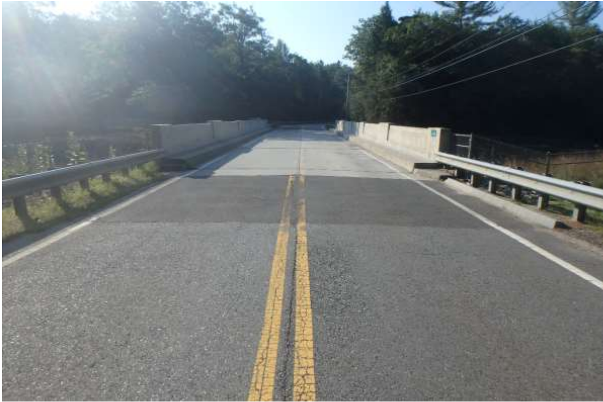
Photo 13: Tully Lake Spillway Bridge – Plan View
