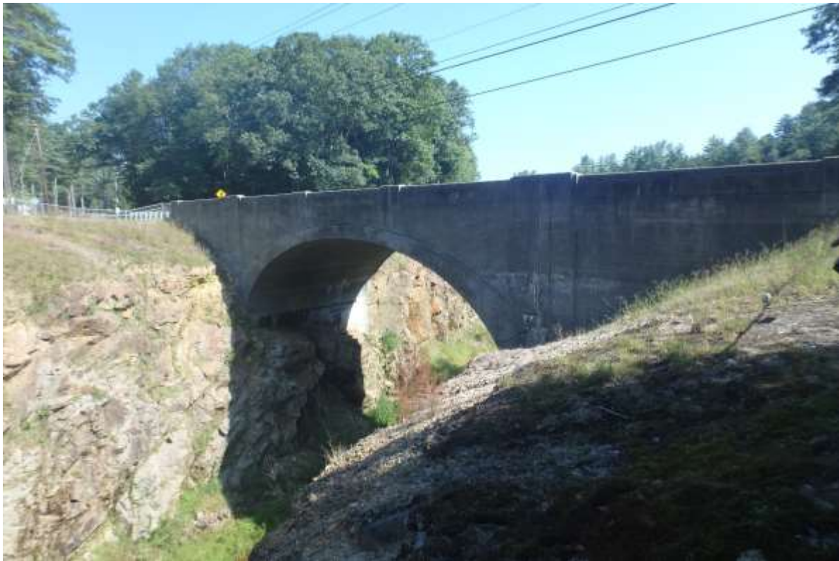
Photo 14: Tully Lake Spillway Bridge – Elevation View
