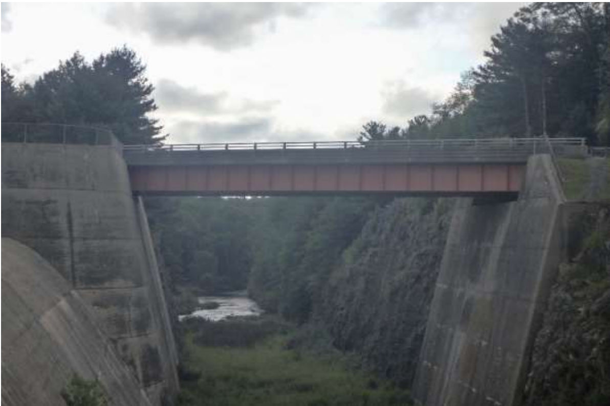
Photo 4: West Thompson Lake Spillway Bridge – Elevation View
