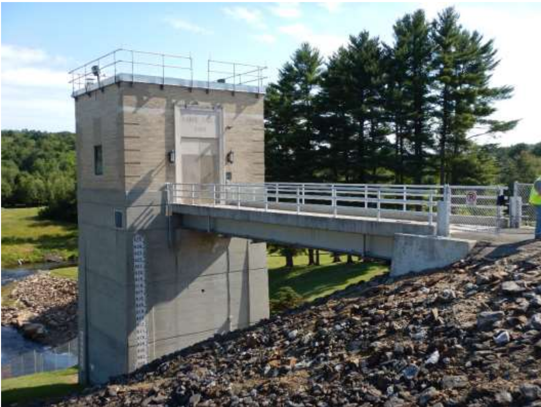
Photo 12: Barre Falls Dam Service Bridge – Elevation View
