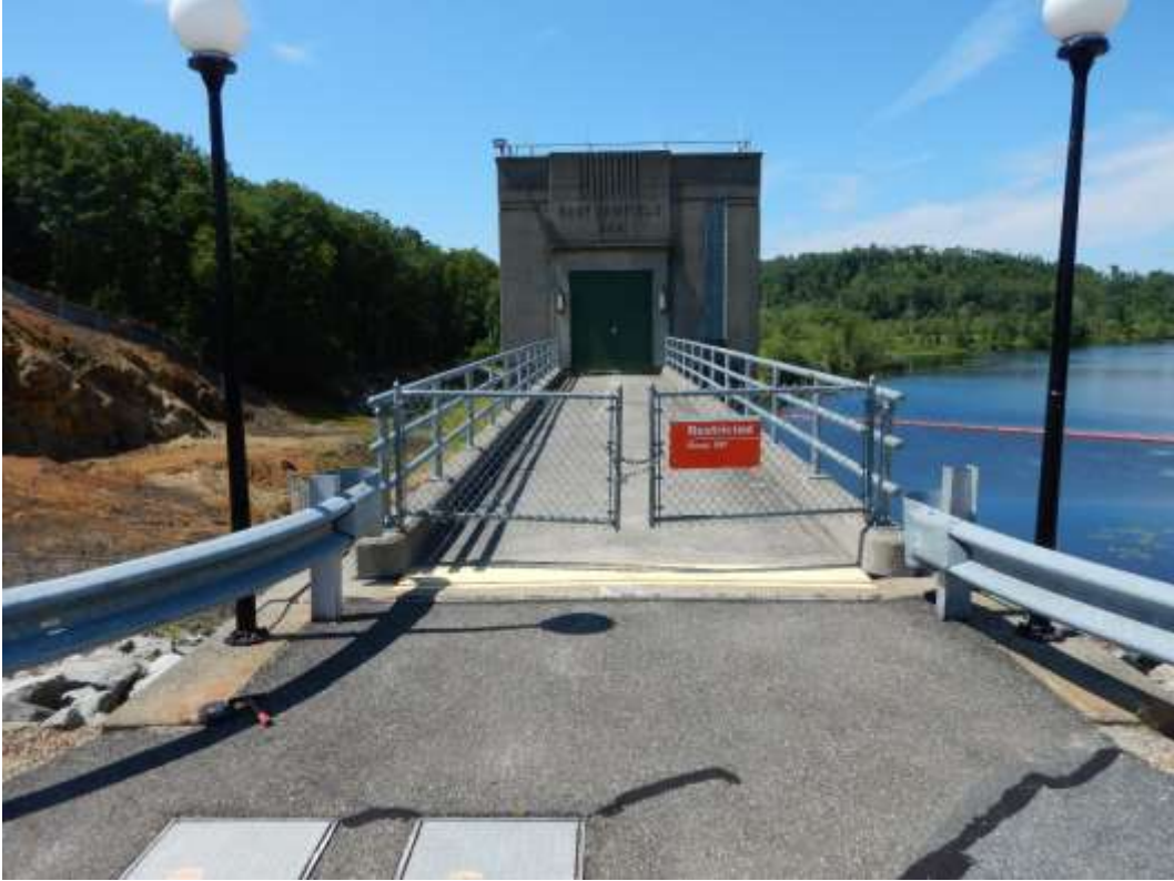
Photo 5: East Brimfield Lake Service Bridge – Plan View
