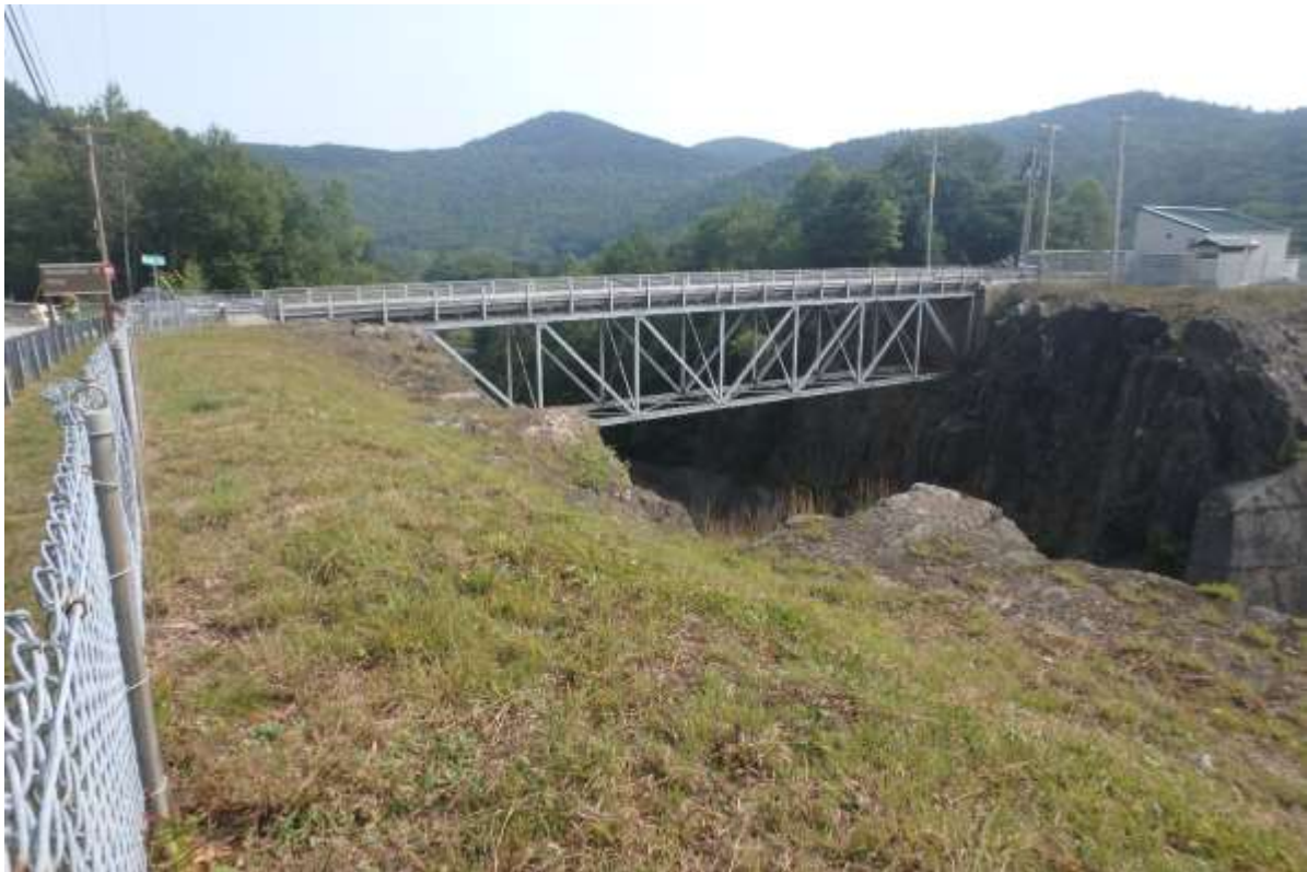
Photo 20: Townsend Lake Spillway Bridge – Elevation View
