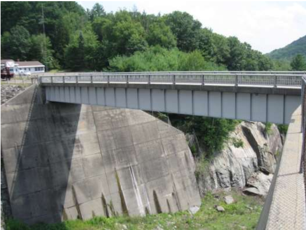
Photo 8: Littleville Lake Spillway Bridge – Elevation View
