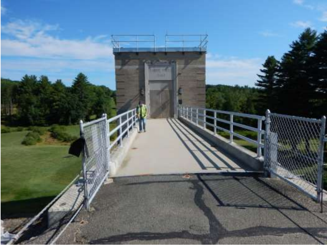
Photo 11: Barre Falls Dam Service Bridge – Plan View
