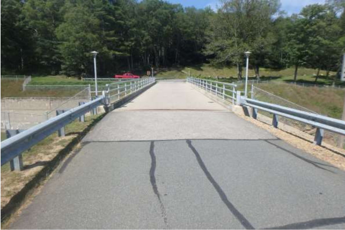
Photo 9: Barre Falls Dam Spillway Bridge – Plan View
