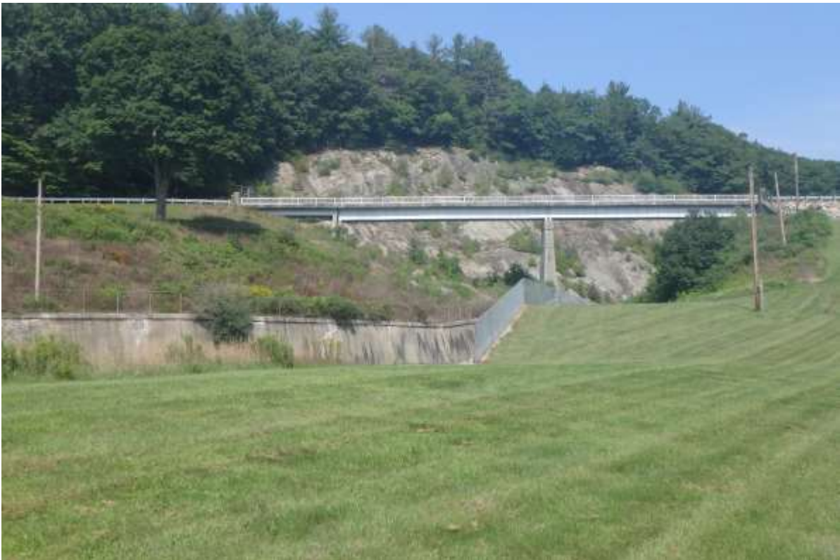
Photo 16: Surry Mountain Lake Spillway Bridge – Elevation View
