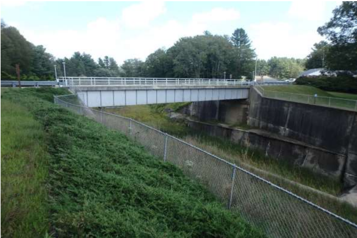
Photo 10: Barre Falls Dam Spillway Bridge – Elevation View
