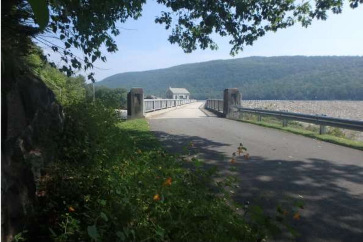
Photo 15: Surry Mountain Lake Spillway Bridge – Plan View
