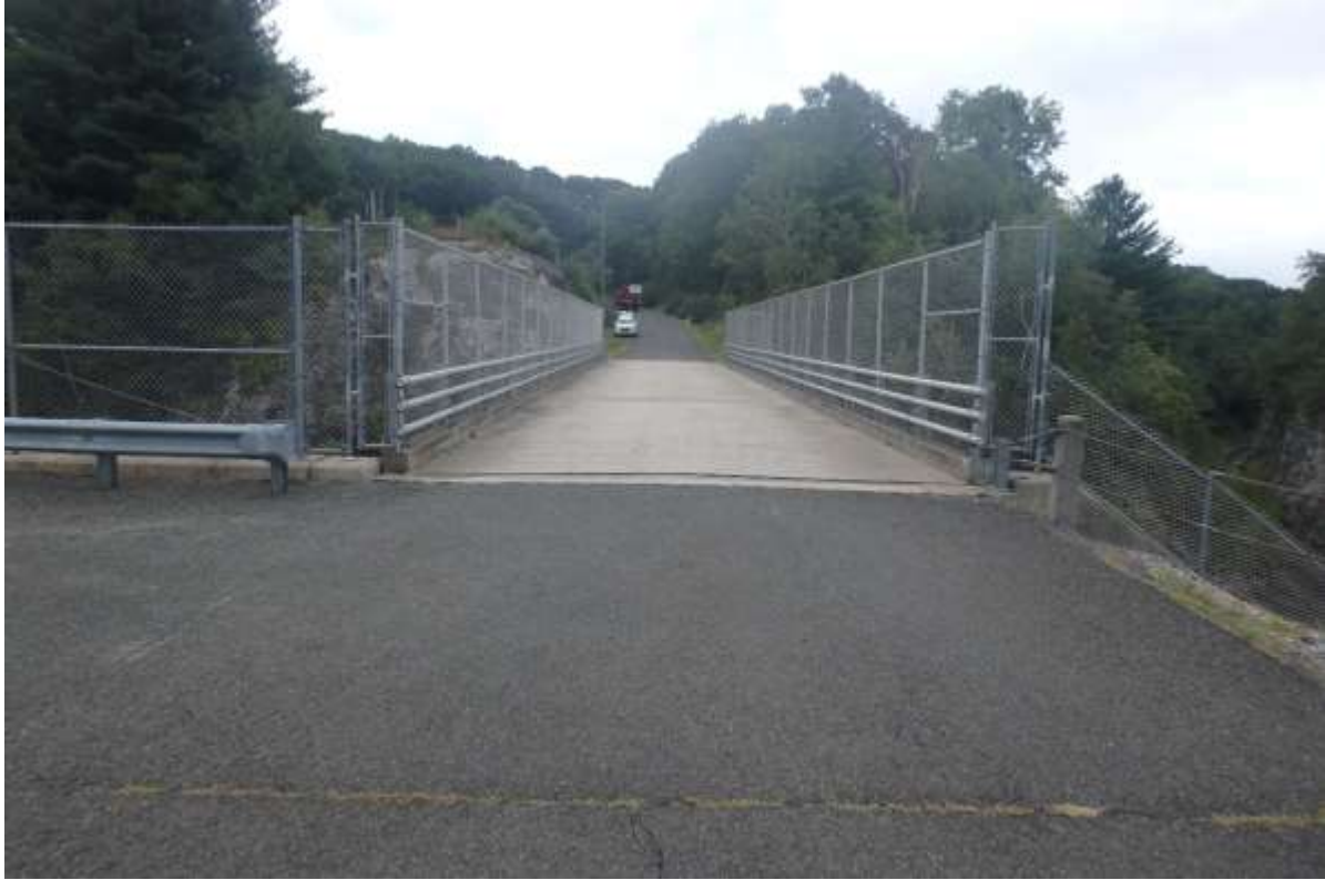
Photo 1: Thomaston Dam Spillway Bridge – Plan View
