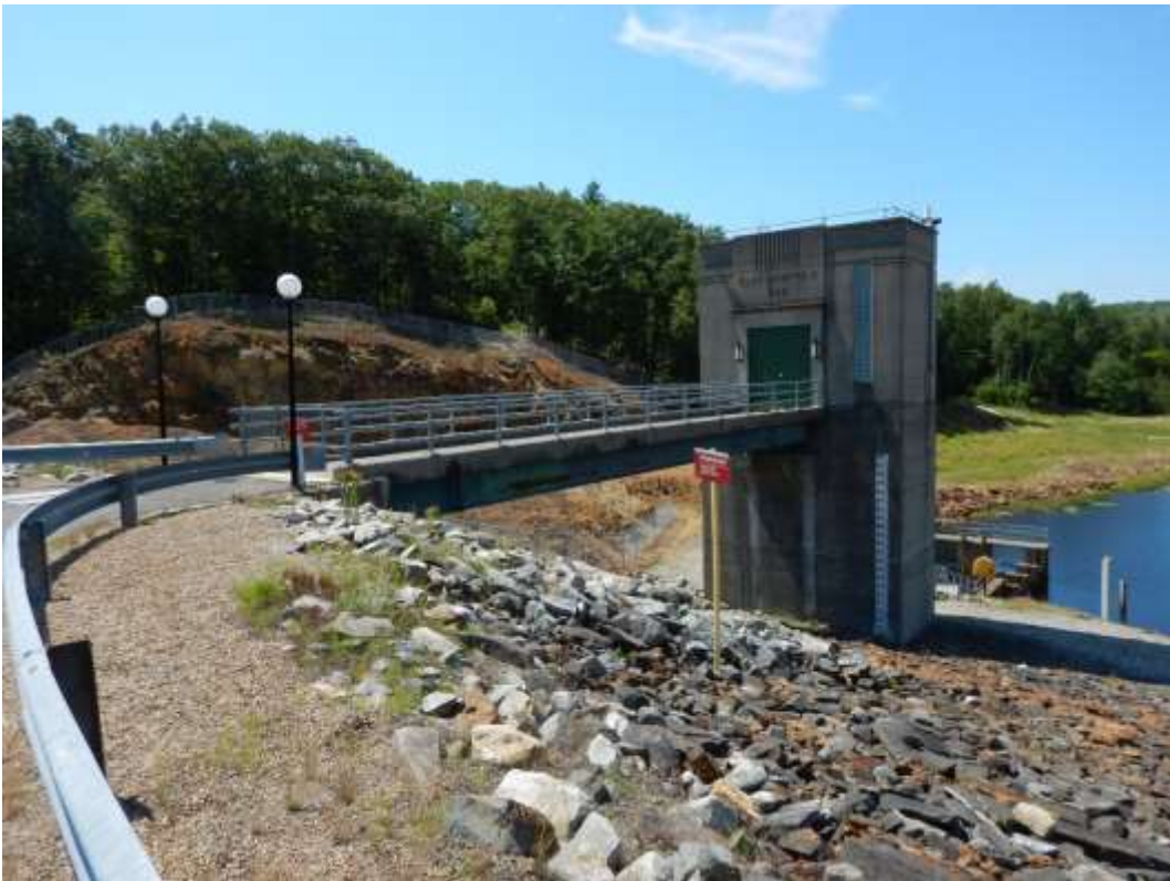
Photo 6: East Brimfield Lake Service Bridge – Elevation View
