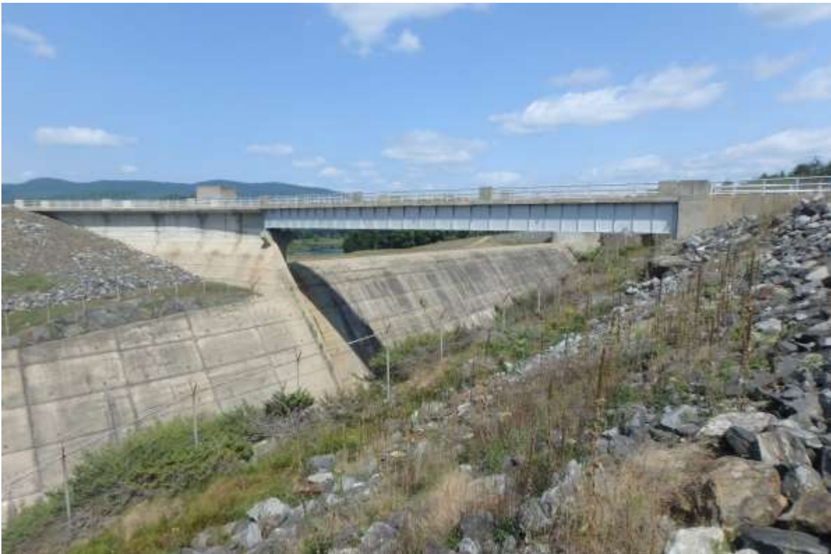
Photo 18: North Springfield Dam Spillway Bridge – Elevation View
