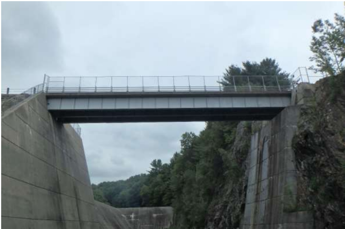
Photo 2: Thomaston Dam Spillway Bridge – Elevation View
