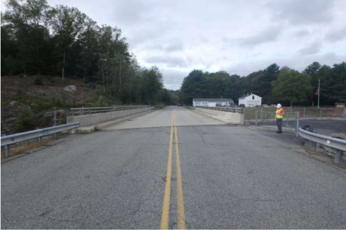
Photo 3: West Thompson Lake Spillway Bridge – Plan View
