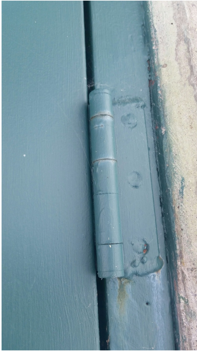
Informational Photos 5 & 6 – Gate house main door hinges outside welded, and inside Philips screw attachment.
