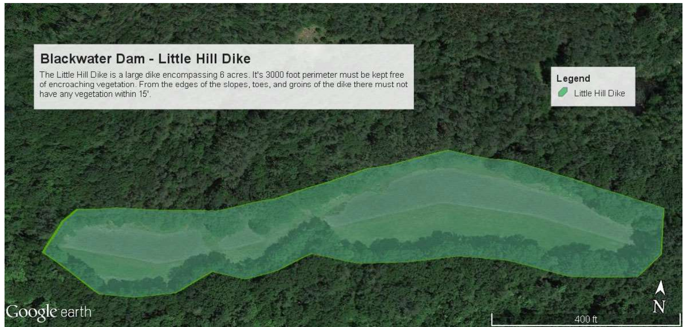
Exhibit D: Vegetation removal around the perimeter of Little Hill Dike.
