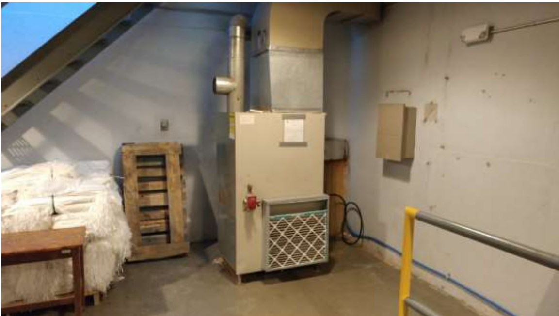
Informational Photo 2: Highboy Furnace to be removed for disposal
