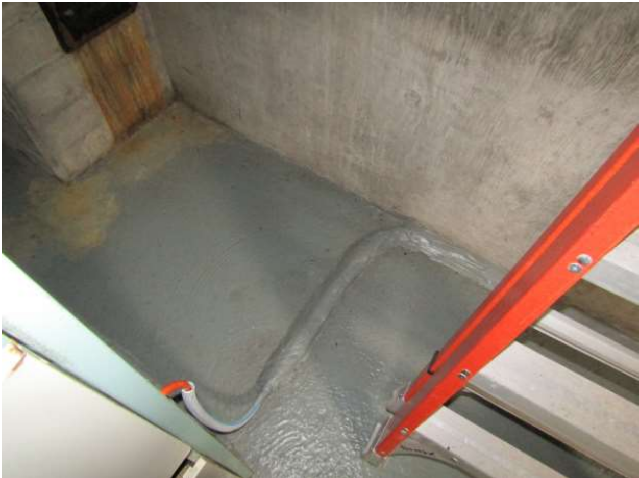
Informational Photo Number 6. Existing fuel lines.
