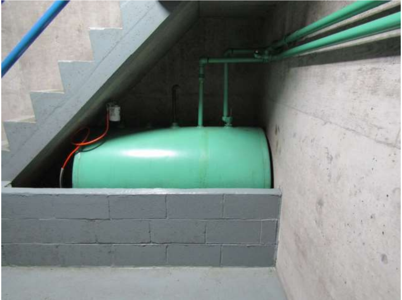
Informational Photo Number 2. Existing 260 gallon NO 2 fuel oil storage tank, masonry secondary containment wall, supply lines, and filter assembly.
