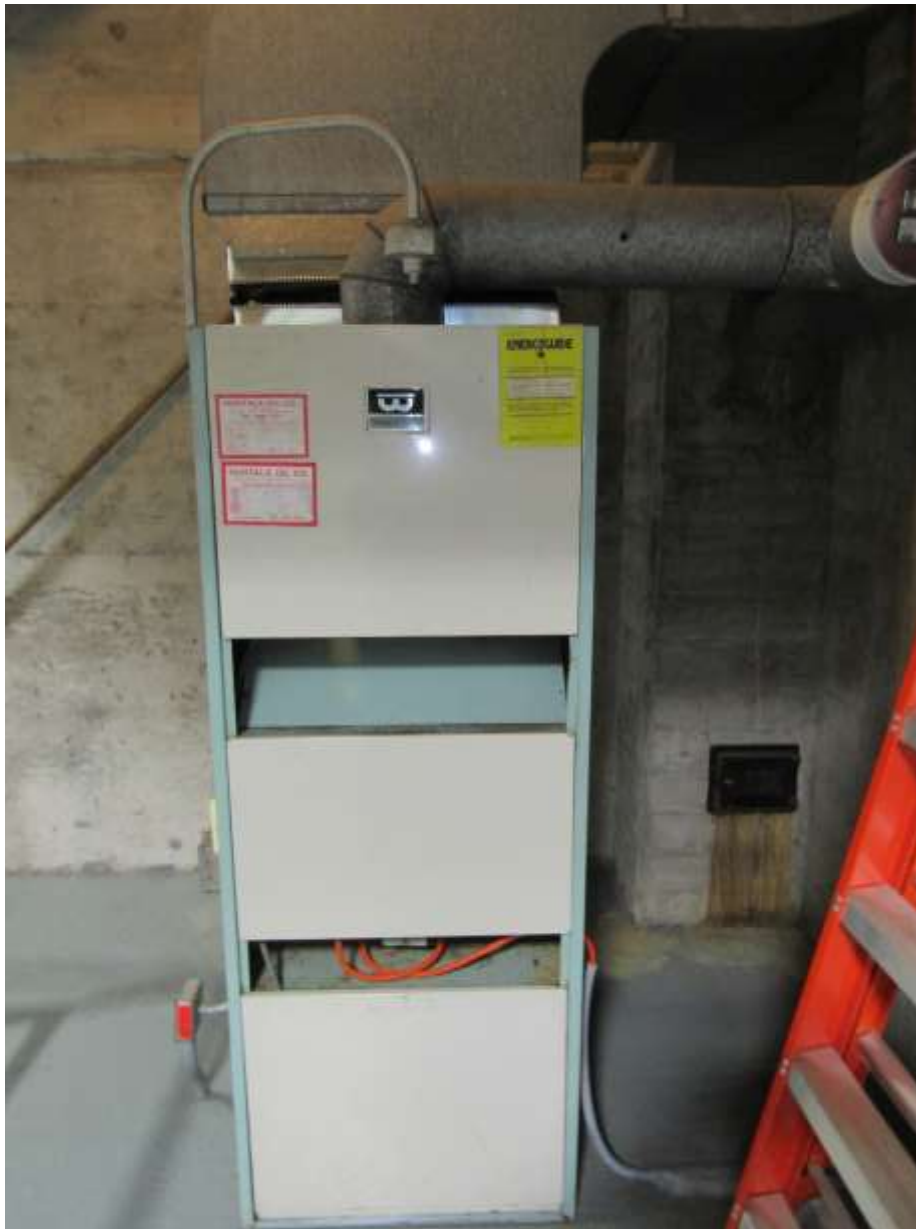
Informational Photo Number 1. Existing Williamson Temp-O-Matic Model 1167-18-1 Warm Air Furnace, supply line, and duct work.
